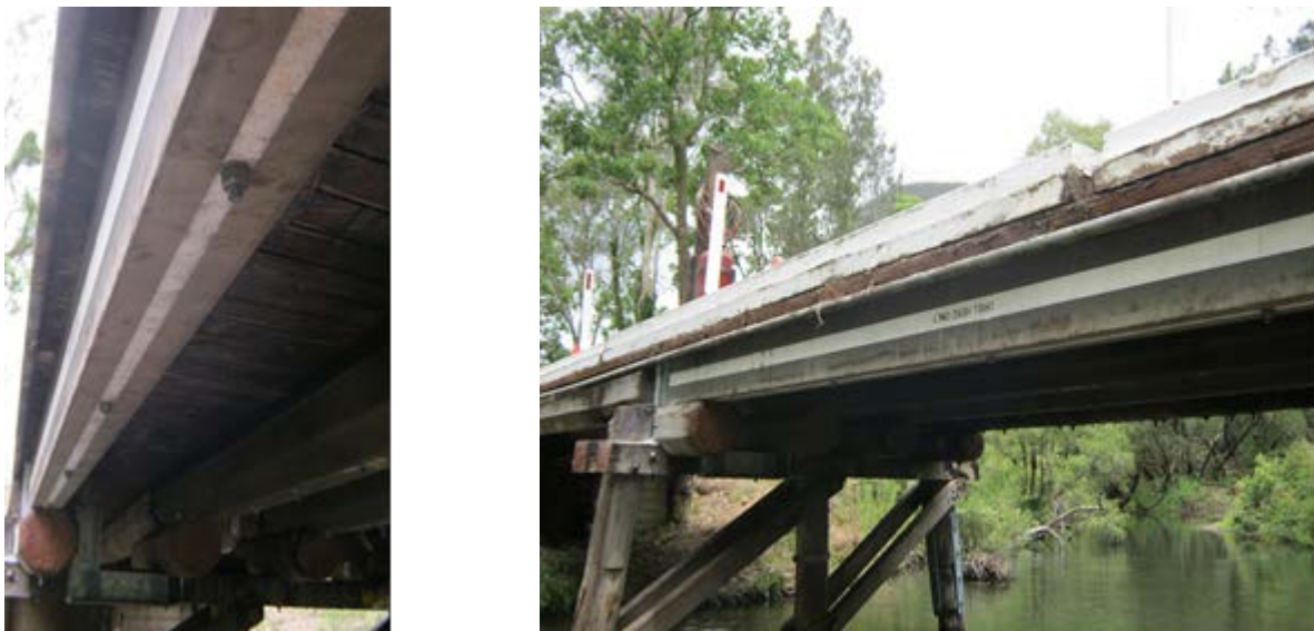
Figure 10.5b - Completed FRPC girder installed on Coulson Creek bridge
