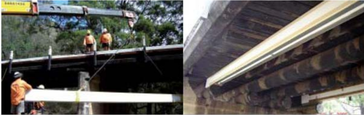
Figure 10.4b - Installation of FCDD girder
