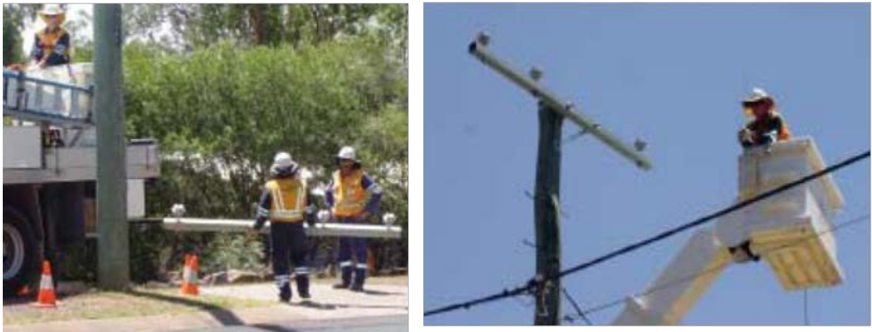
Figure 5a - Wagners CFT cross-arm installation
