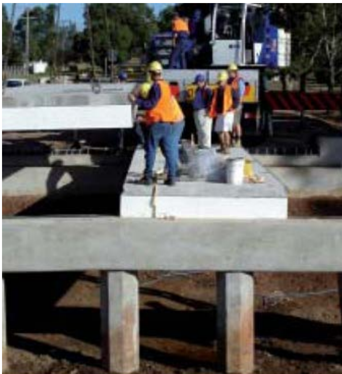
Figure 11.2a - Wagners CFT bridge installation
