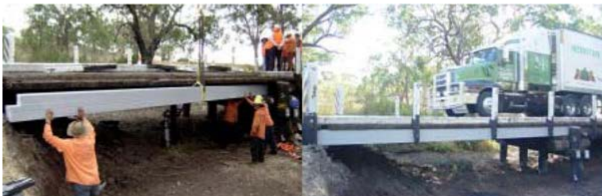
Figure 10.3b - Beam installation and working under load
