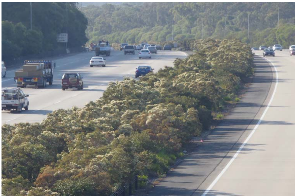
Figure A3-15: The maintenance interventions of planted median will progressively reduce to one intervention per annum
