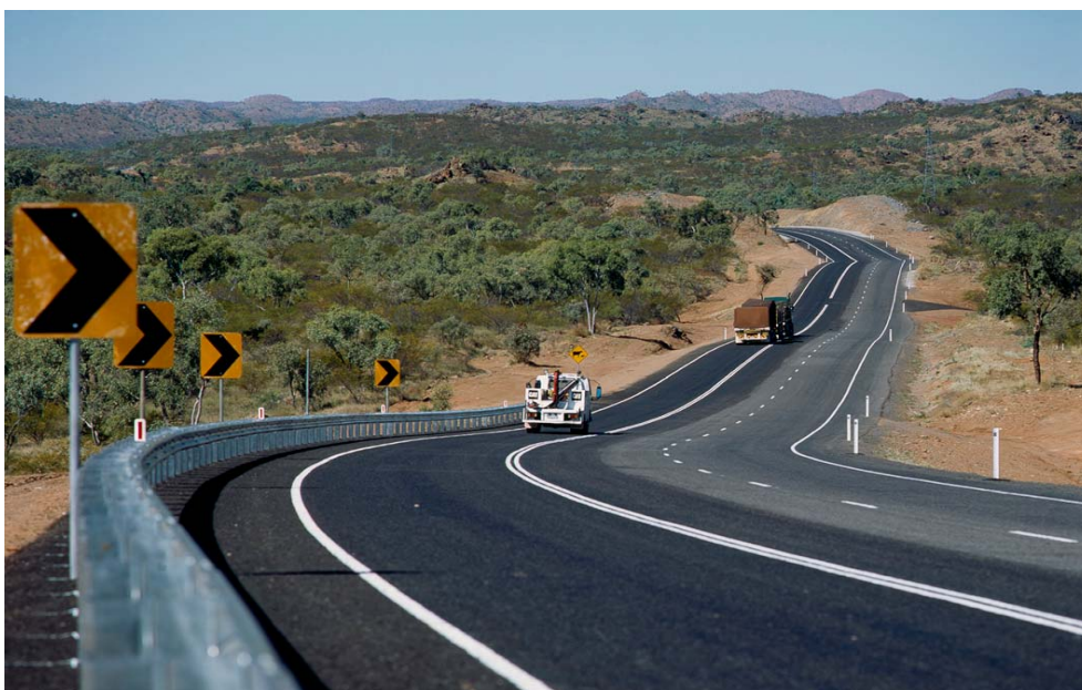
Figure A3-3: Barkly Highway between Cloncurry and Mt Isa
