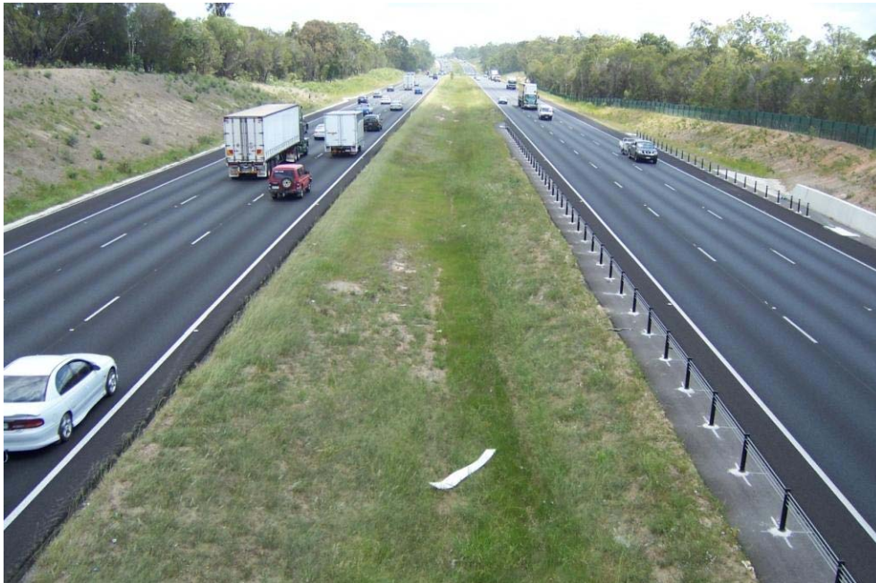
Figure A3-14: Slashing/ mowing to grassed median and verge requires 8 to 10 maintenance interventions per annum
