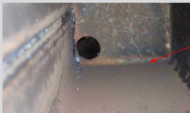
Figure 8.5.4(b) – View of the full penetration butt weld
