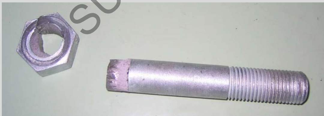
Figure 7.3 – Abnormal bolt failure
