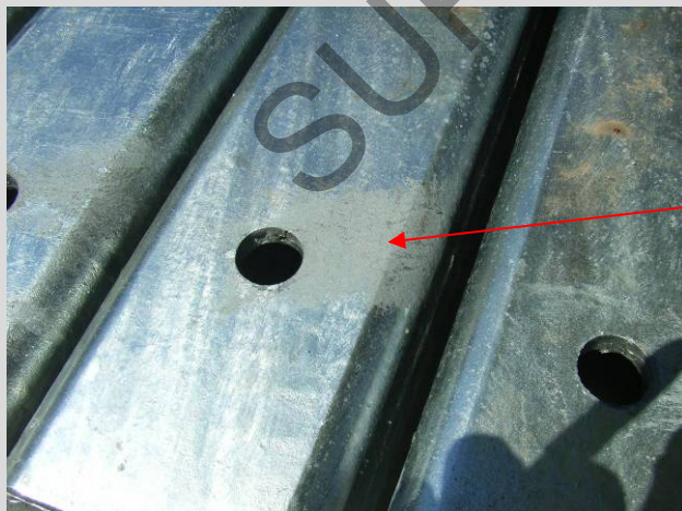
Figure 11.3.3 – View of the zinc rich paint repair
