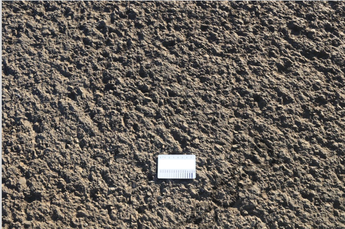
Figure 8.9.9.4.2(b) – Example of an acceptable hard-cut surface
