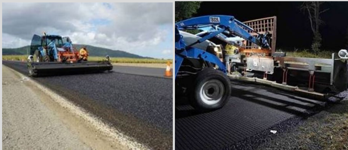
Figure 9.4.2(a) – Examples of installation of asphalt geosynthetics using application frame
