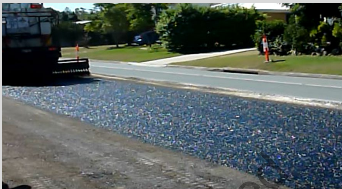
Figure 9.3.3(a) – Example of C170 bitumen bond sprayed on a prepared pavement surface
