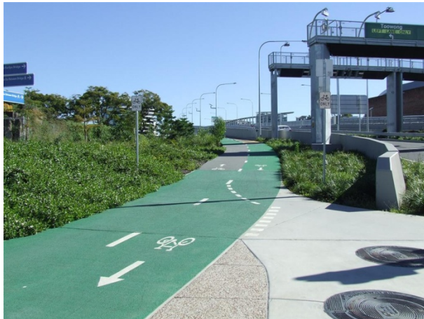
(c) Go-Between Bridge (cycleway)
