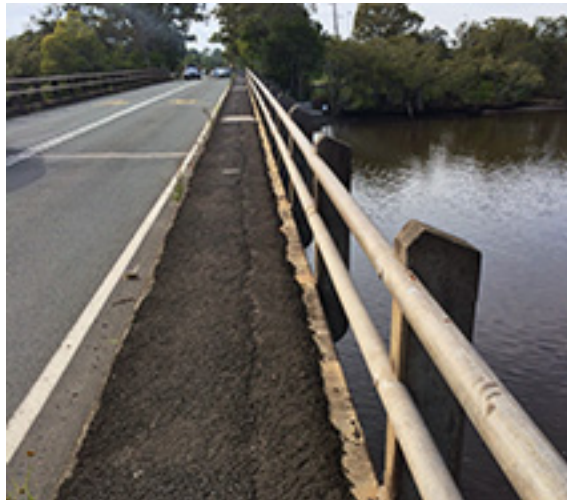
(a) Footpath on south side of road bridge
