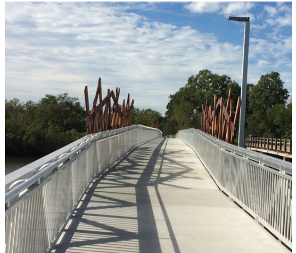
(b) Pedestrian and cyclist bridge
