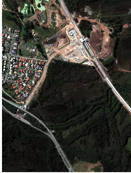
Aerial Image at Rothwell Station (15/04/2015)
