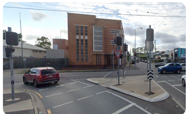
Figure 2: Signalised slip lane
