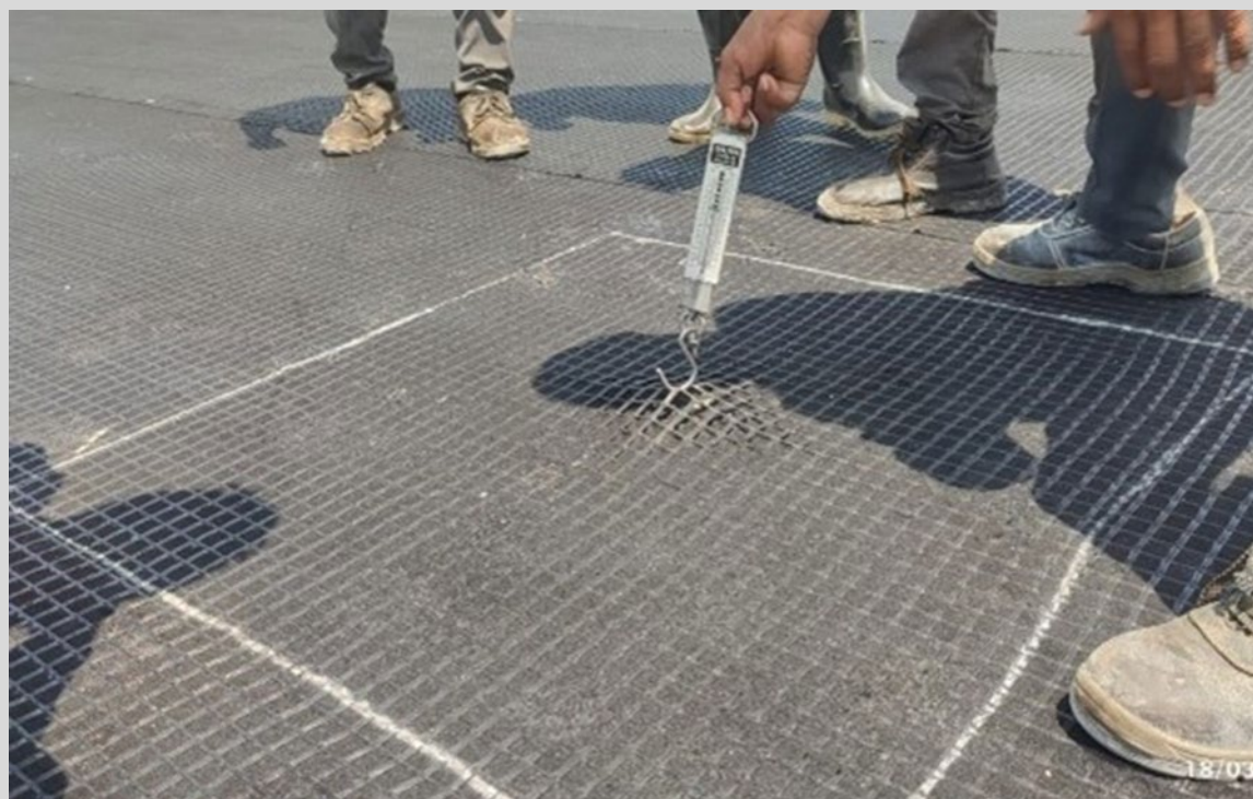
Figure 10.2.5 – Spring balance test to measure the construction bond strength
