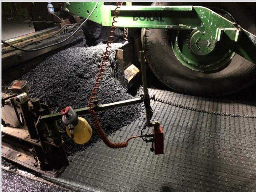
Figure 9.7.1 – Asphalt being paved on asphalt geosynthetic with no bow-waves, wrinkles or folds
