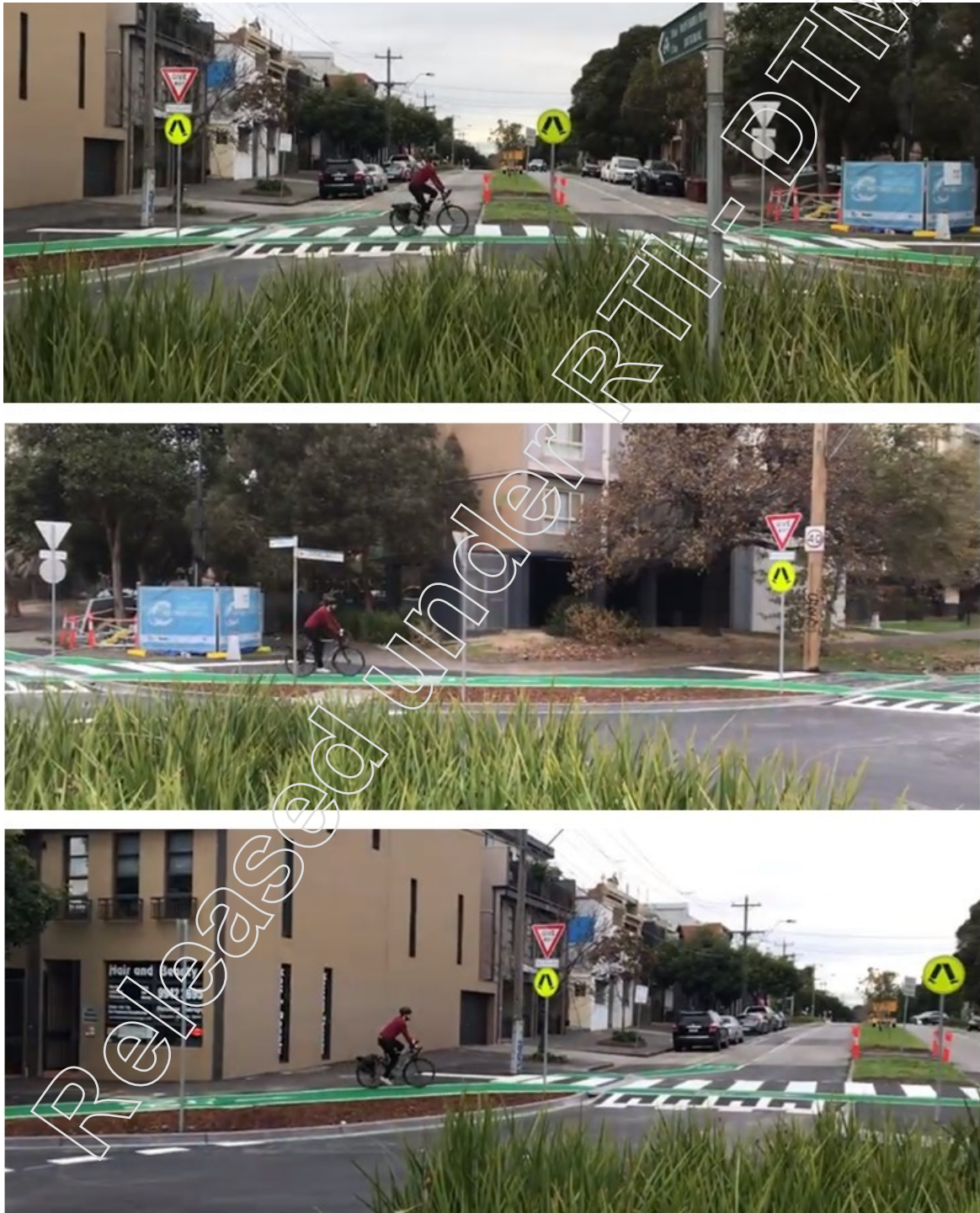
Figure 2.6.4(a) – Raised crossings at roundabout on Moray and Dorcas Street, South Melbourne
