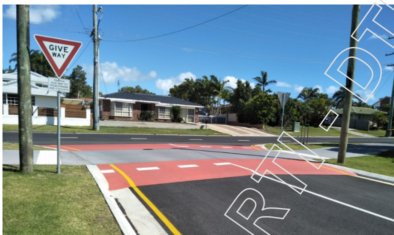
Figure 1.1 – Example of a raised priority crossing for a shared pathway, Mooloolaba Qld
