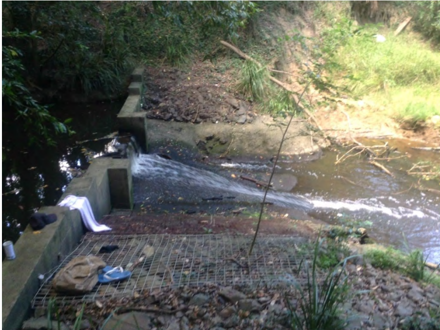
Plate 3-4 Weir constructed within the Deep Creek upstream reach
