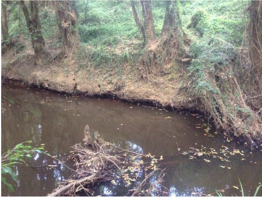
Plate 3-3 Exposed roots and undercut banks along Six Mile Creek
