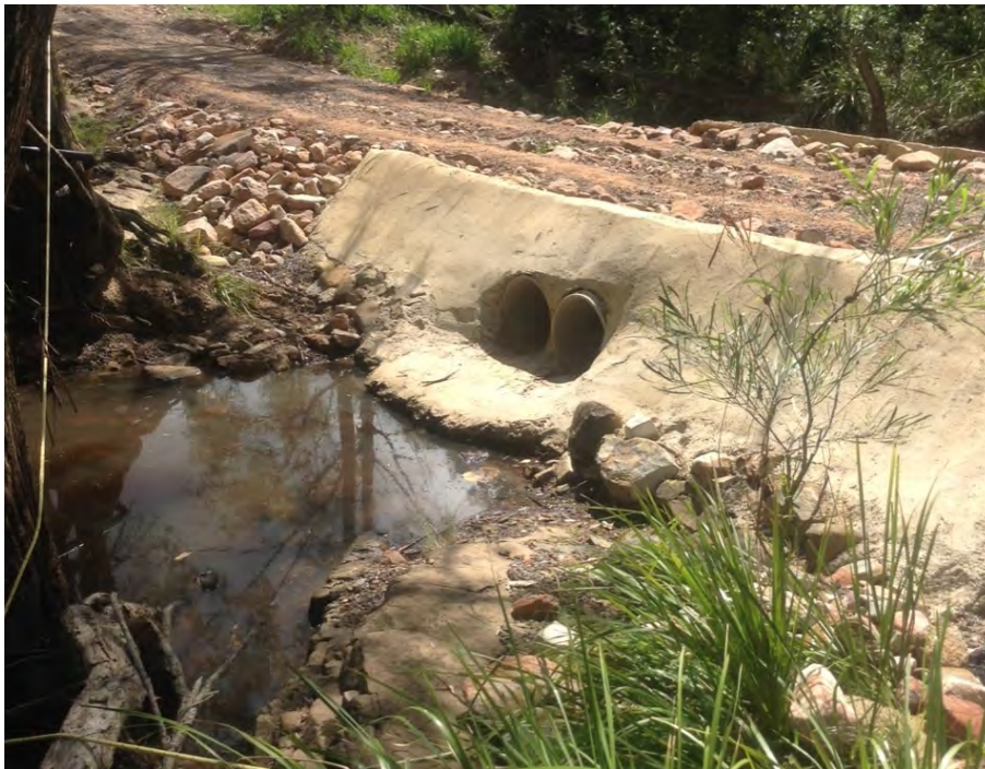
Plate 3-9 Piped culvert on Curra Creek causing fish barrier under low flow conditions
