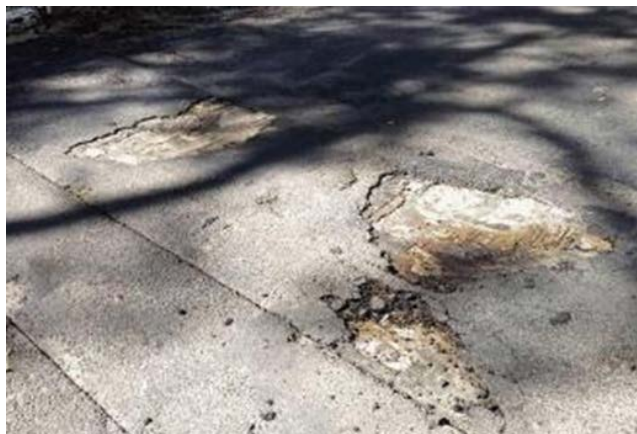
Figure 3.3.3.2a – Abrasion of wearing surface
