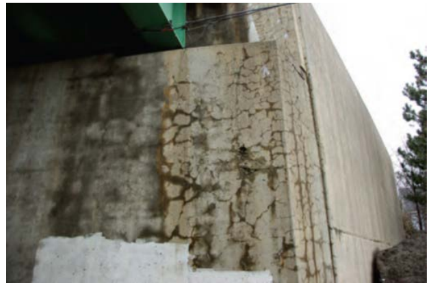
Figure 2.2.2d – Example ASR crack pattern in prestressed deck unit soffit
