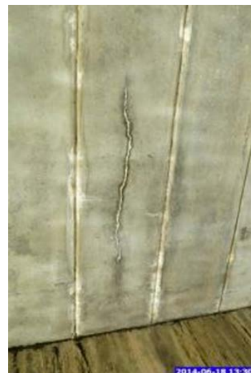
Figure 2.2.2d – Example ASR crack pattern in prestressed deck unit soffit
