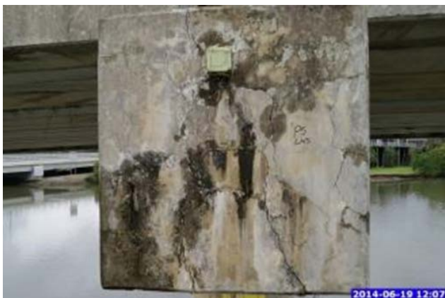
Figure 2.2.2c – Example ASR crack pattern in pier headstock
