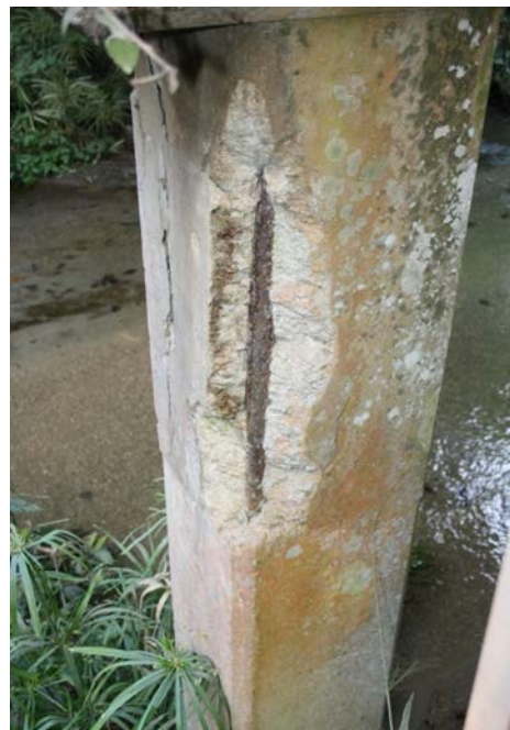
Figure 2.2.4d – Corner spalling of square pile
