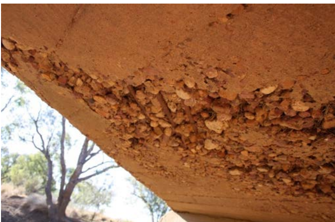
Figure 2.2.6e – Concrete honeycombing
