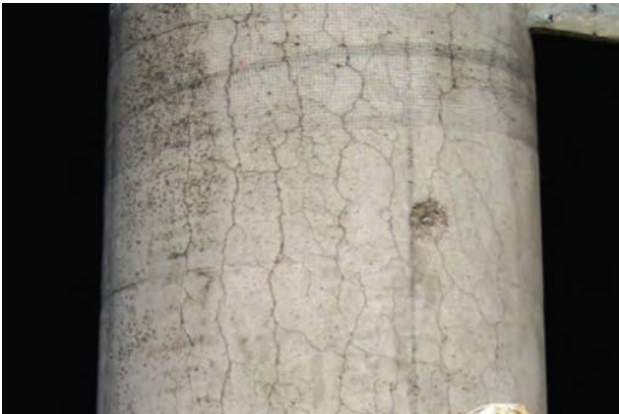
Figure 2.2.2c – Example ASR crack pattern in pier headstock
