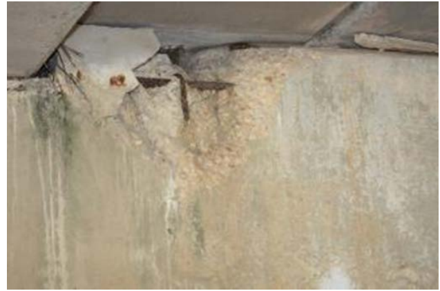
Figure 2.2.4d – Corner spalling of square pile
