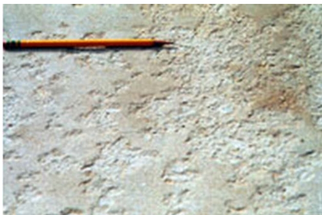
Figure 2.2.7a – Concrete scaling
