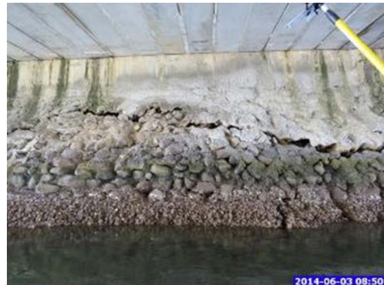
Figure 3.5.7d – Settlement of rigid batter protection
