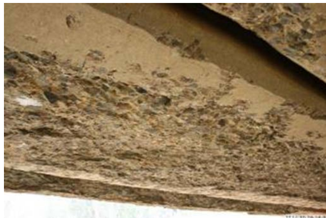
Figure 2.2.7b – Concrete disintegration
