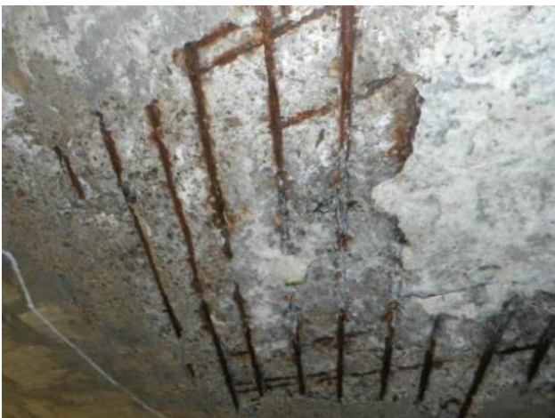
Figure 2.2.4c – Spalling of slab soffit
