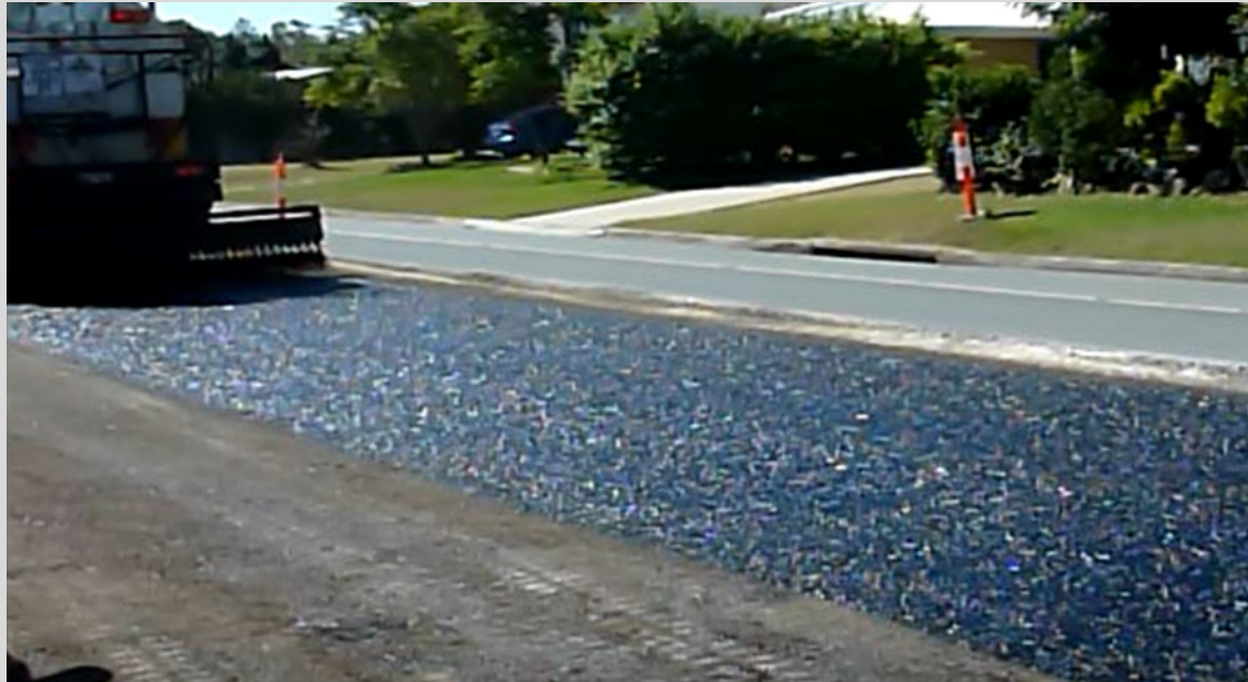
Figure 8.6.2 – C170 bitumen bond coat being sprayed on a prepared pavement surface
