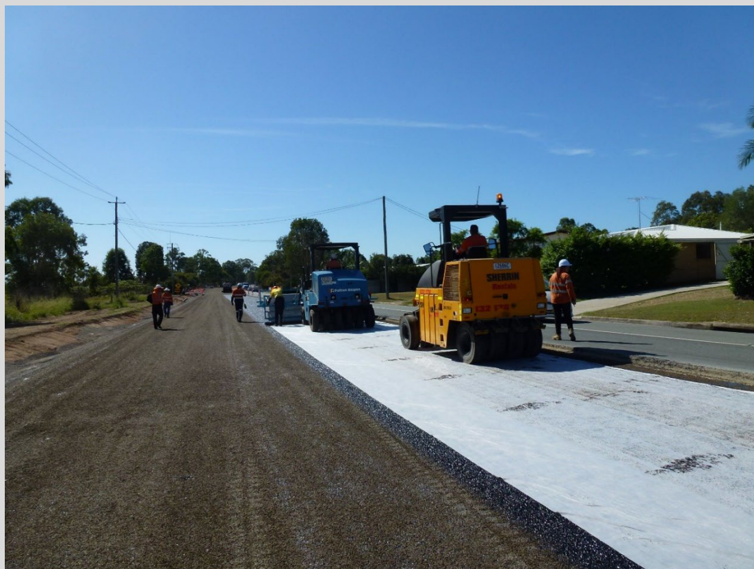
Figure 8.7.2 – Installation of geotextile using application frame attached to multi-tyred roller
