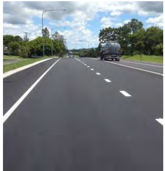
An example of asphalt surface
