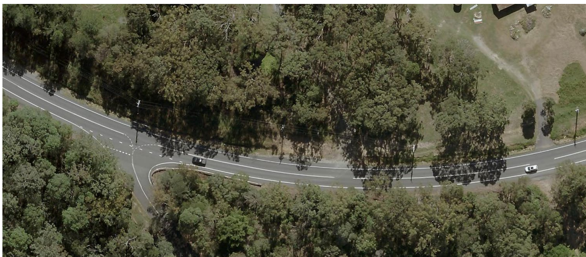
Figure A1 – Features of the Redland Bay Road / Riedel Road intersection, Carbrook
