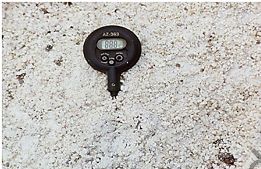
Figure 8.6.6.2.3 – Checking completion of slaking with temperature probe
