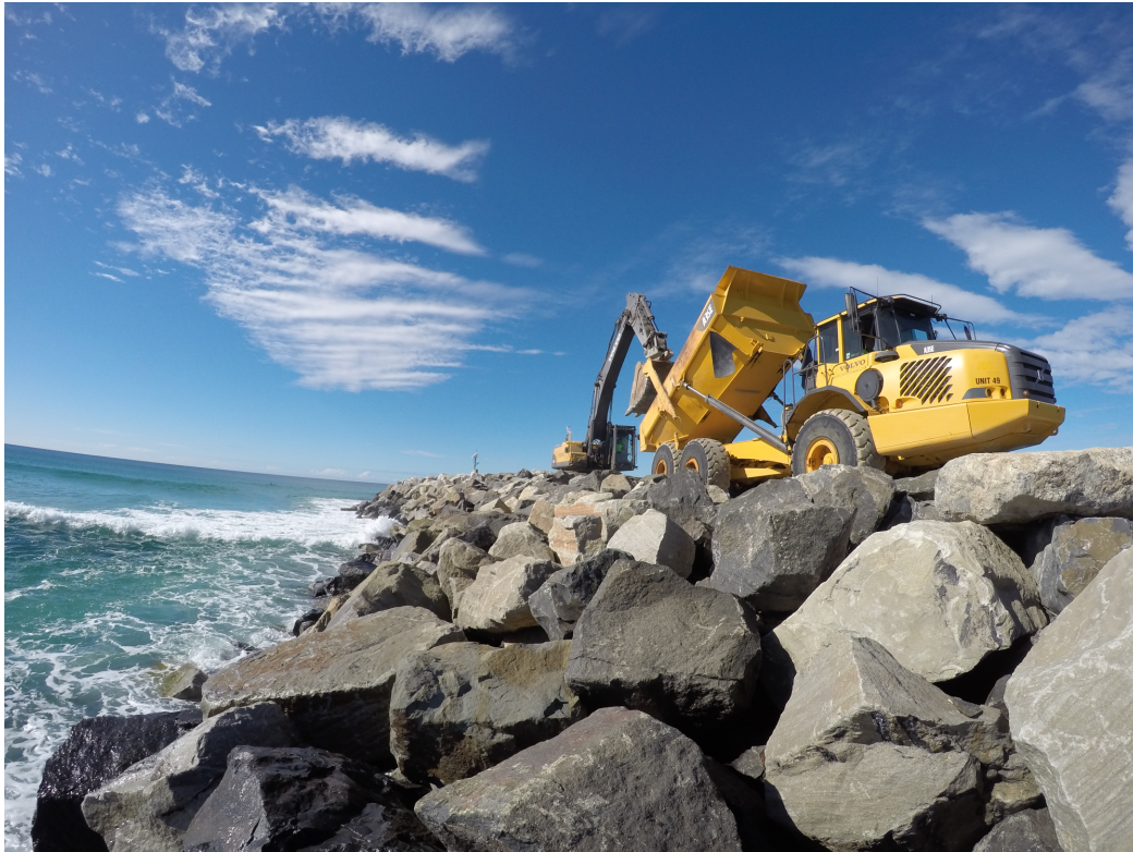
Figure 7 – 35T Articulated Dump Truck Unloading Armour Rock at Brunswick Heads Breakwater
