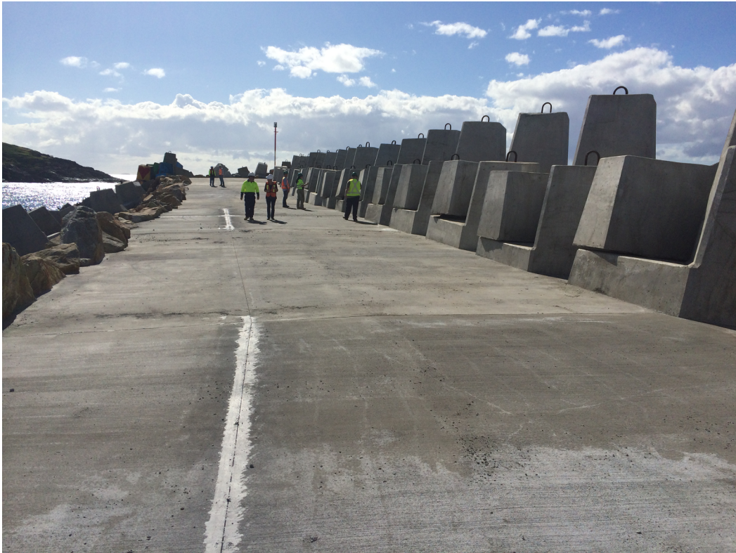
Figure 16 - Concrete Pavement Coffs Harbour Eastern Breakwater
