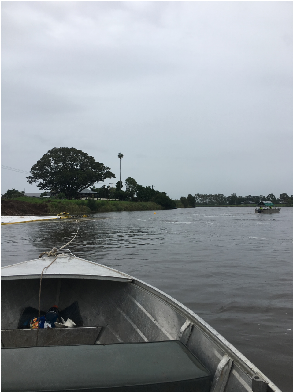
Figure 2 - Divers assisting in placing 600R geotextile (Nelsons Plains)
