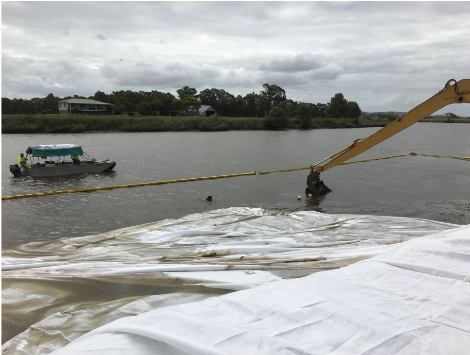
Figure 3 - Divers and excavator placing 600R geotextile (Nelsons Plains)
