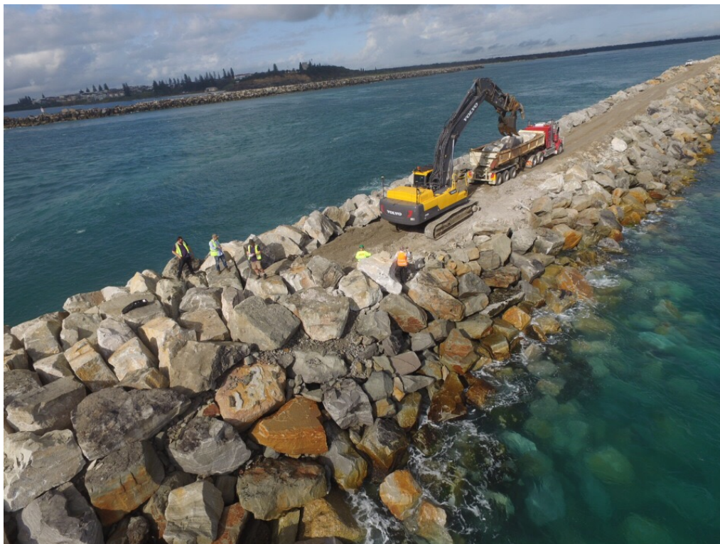
Figure 5 - Side Tipper Carting Rock to Iluka Breakwater
