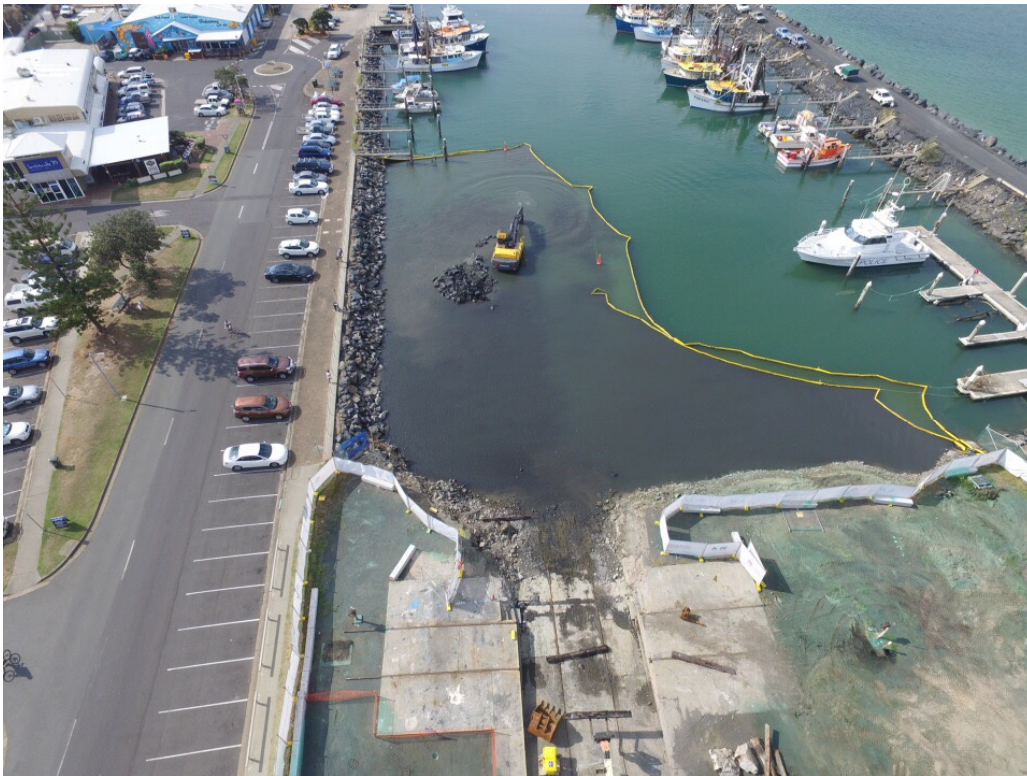
Figure 17 - Maintenance Dredging Coffs Harbour Marina
