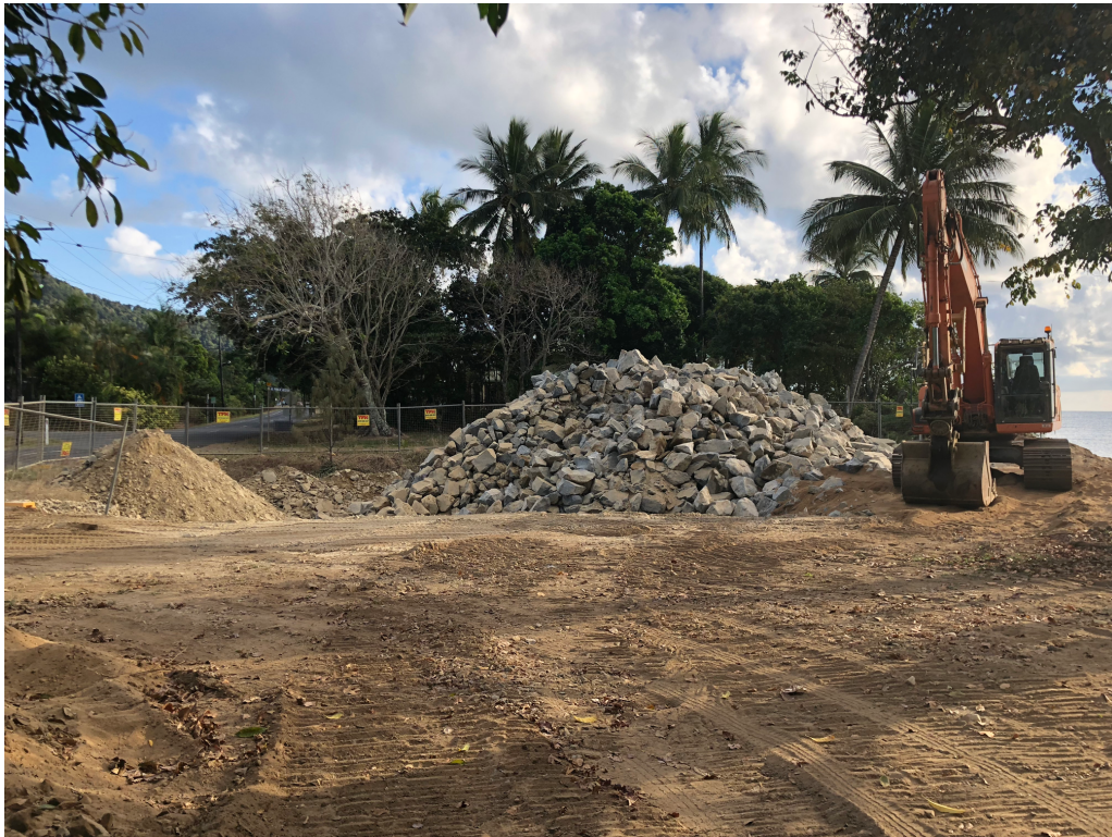
Figure 6 - Filter Rock Stockpile at Flying Fish Point
