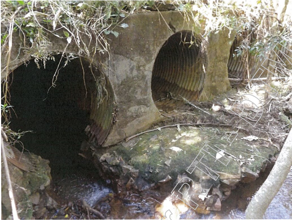
Plate 1 Condition of Existing Culverts
