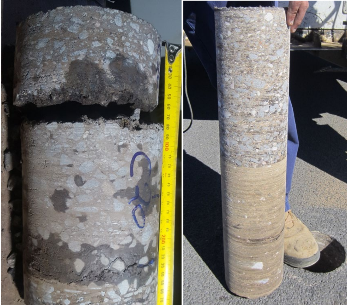
Figure 4.4.2 – Example of 150 mm diameter core of asphalt (left) and stabilised pavement layers (right)
