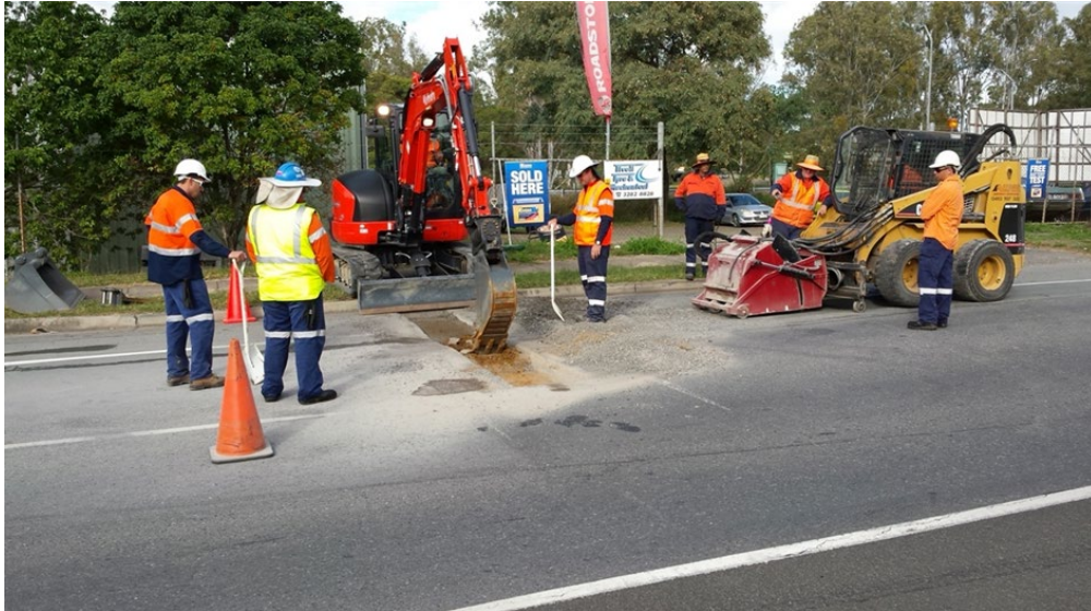
Figure 4.4.4(a) – Example of trenching using excavator with a bobcat milling attachment
