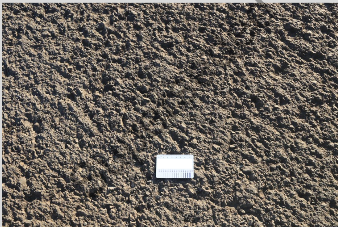
Figure 8.8.9.4.2(b) – Example of an acceptable hard-cut surface
