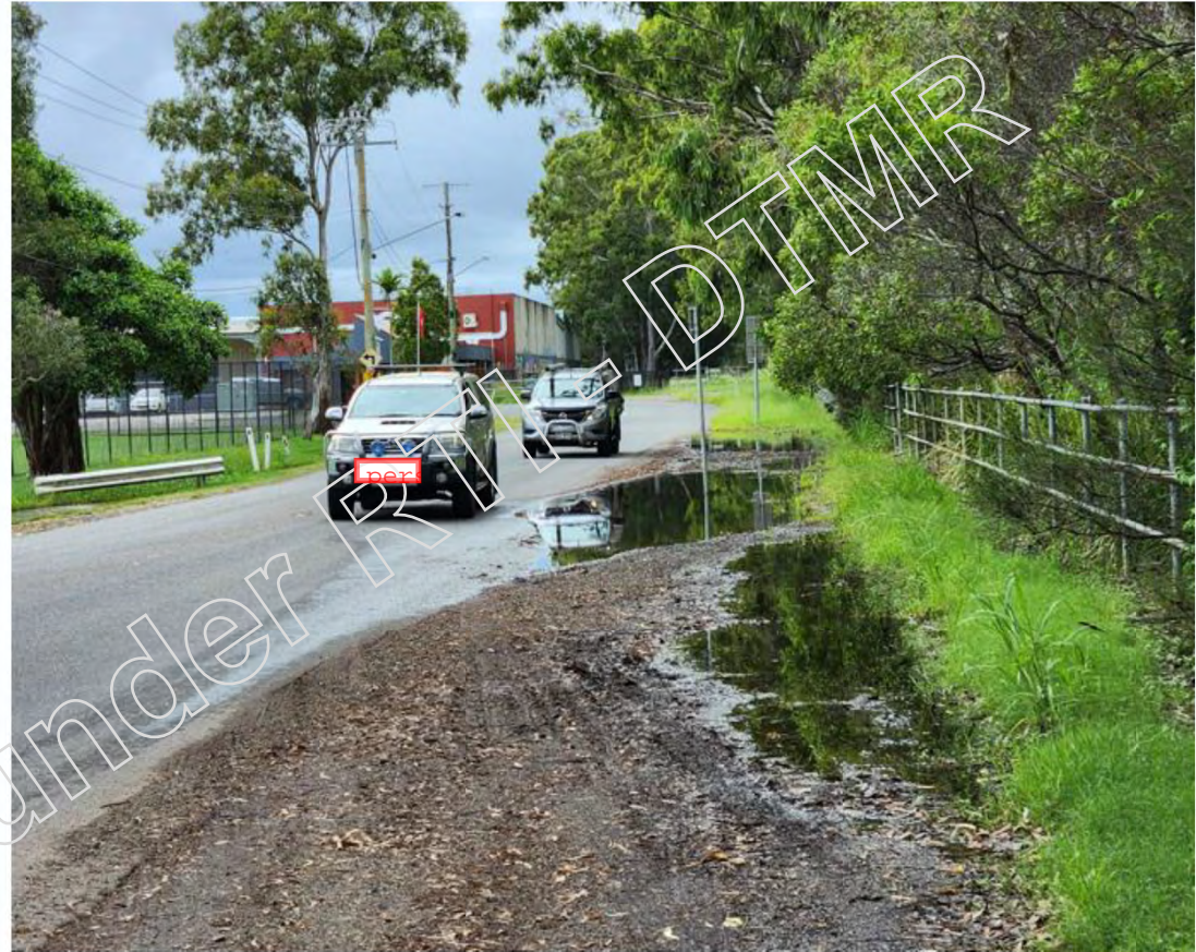
Water level along Sandy Camp Rd worries me. Water ponding at the North Rd bend, looks like it doesn't take much for the roadway to flood due to the adjacent wetland.
