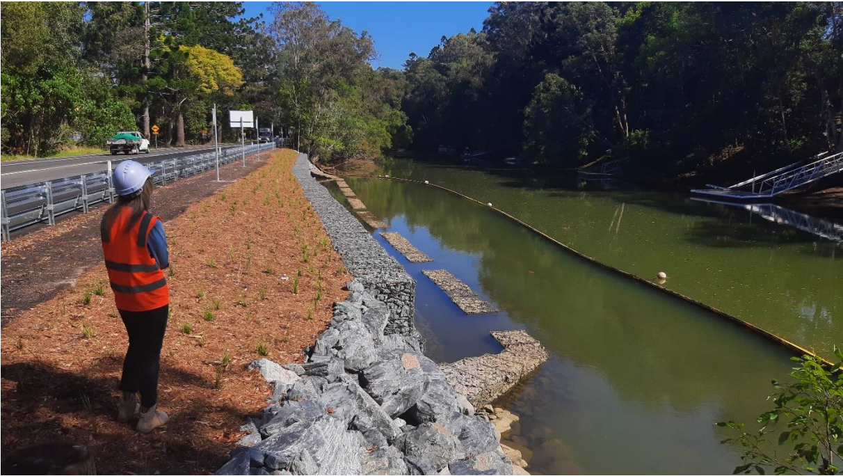
Picture 4 - Completed restoration works on Currumbin Creek Road Site 2 Source: TMR
