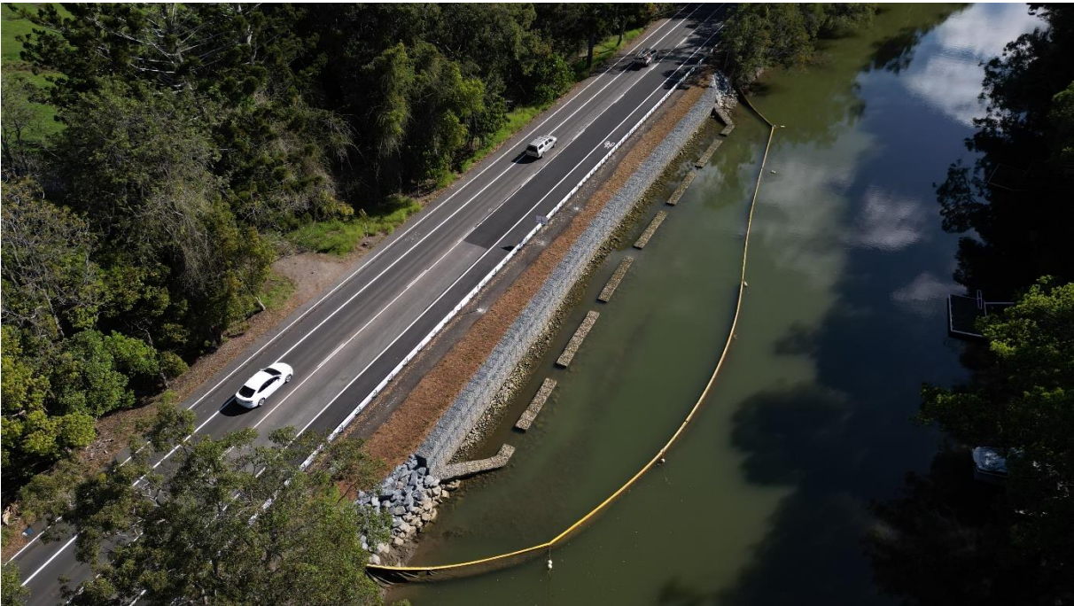
Picture 3 - Completed restoration works on Currumbin Creek Road Site 2 Source: TMR
