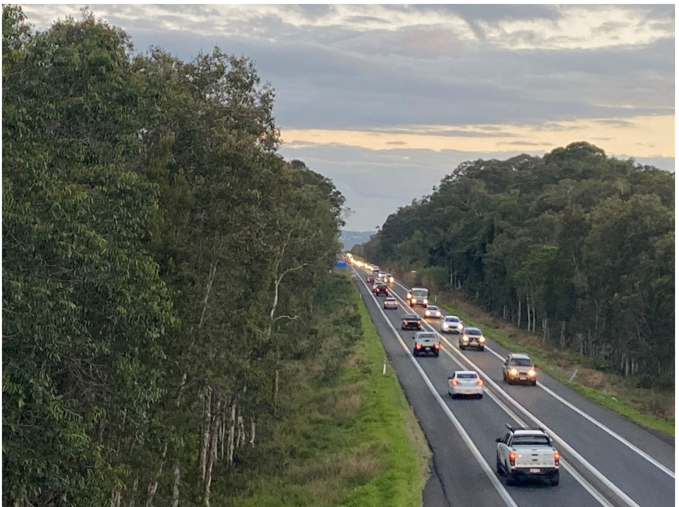
Image: TMR – Sunshine Motorway, south of Coolum.
