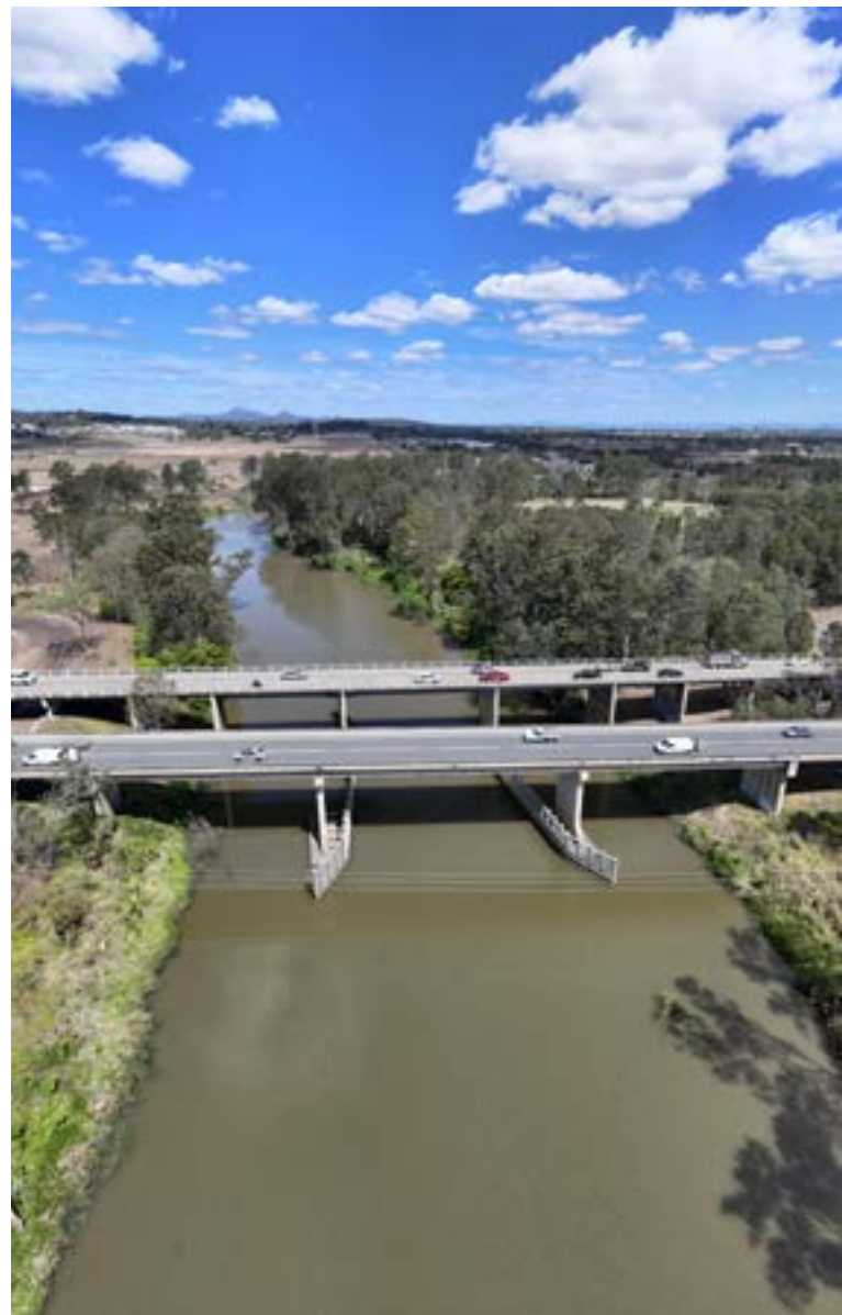
Bremer River Bridge
