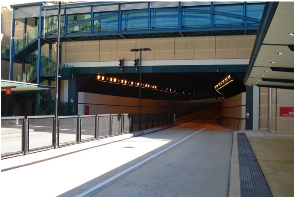
Figure C3-3: A functional and aesthetic tunnel portal through colour and material selection
