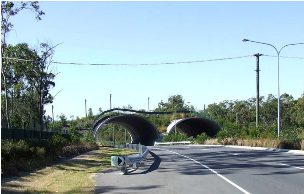
Figure C6-10: Connecting habitat areas through fauna movement devices integrated within the road landscape
