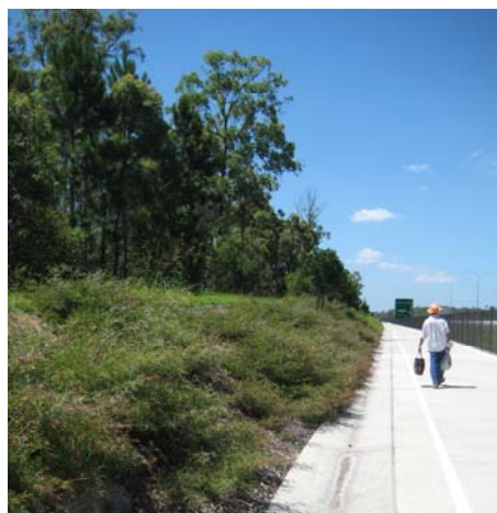
Figure APX4-2: The existing urban forest in the background of this transport and road corridor has been protected for its ecological value
