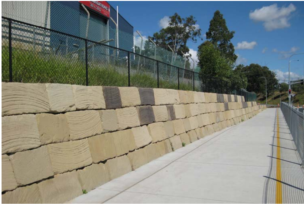
Figure C6-2: Locally sourced stone used in wall, reduces transportation and haulage requirements
