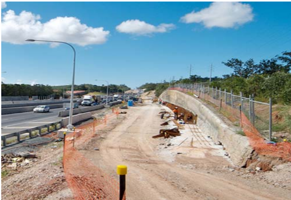
Figure C6-5: Protecting environment from disturbance through limiting footprint
