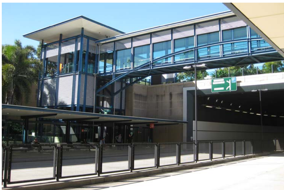
Figure C5-4: Improved surveillance through well designed useable and clearly defined space
