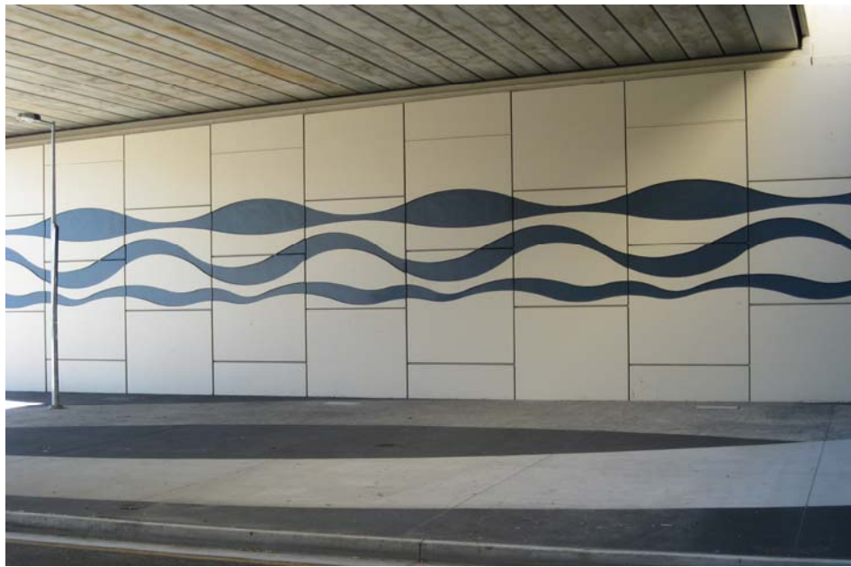
Figure APX2-20: An example of a feature vision implemented through the urban design treatment to the retaining walls of this underpass structure within a new transport and road proposal
