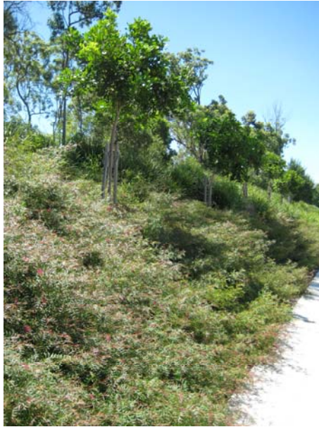
Figure D1-2: Photographic records reflect the standard of installed treatments.
