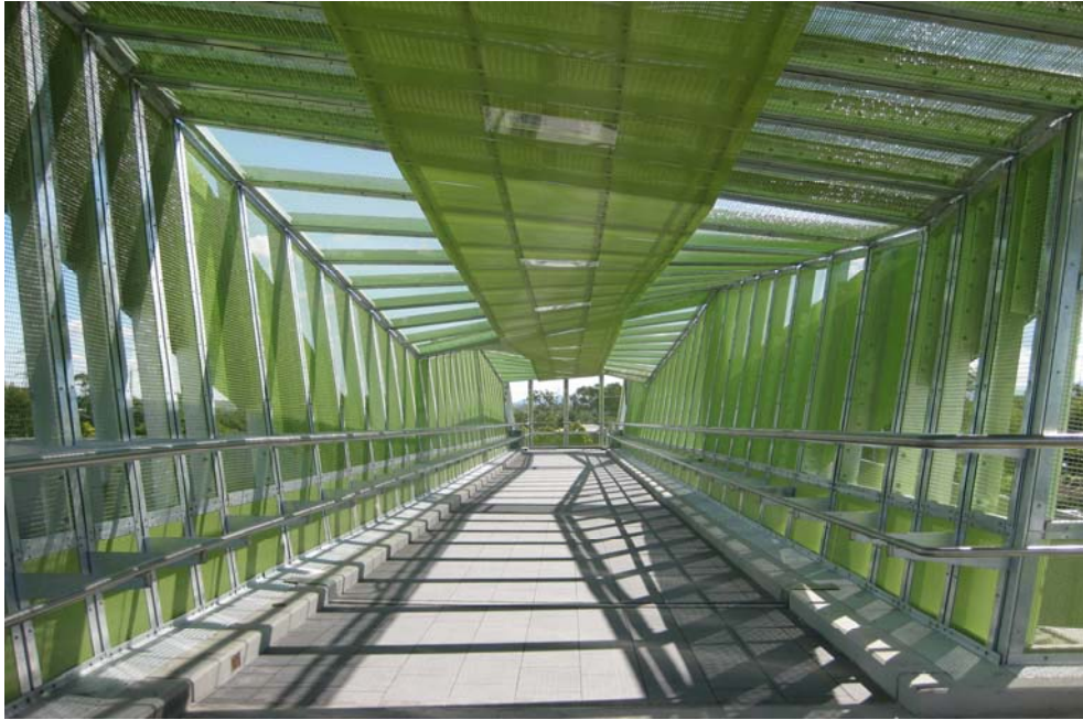
Figure C7-6: Connectivity through pedestrian/cyclist access bridges to public transportation systems is a basic community need within transport and road corridors
