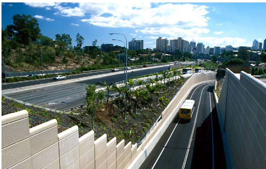
Figure B3-2: Major Projects, such as busways, require a full Integrated Landscape Assessment Report to be produced, due to potential magnitude of impacts on surrounding landscape, particularly in urban areas
