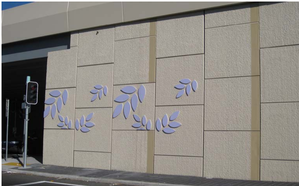
Figure C3-8: Colour and pattern in conjunction with three dimensional art used in retaining wall design to create visual interest and express corridor themes
