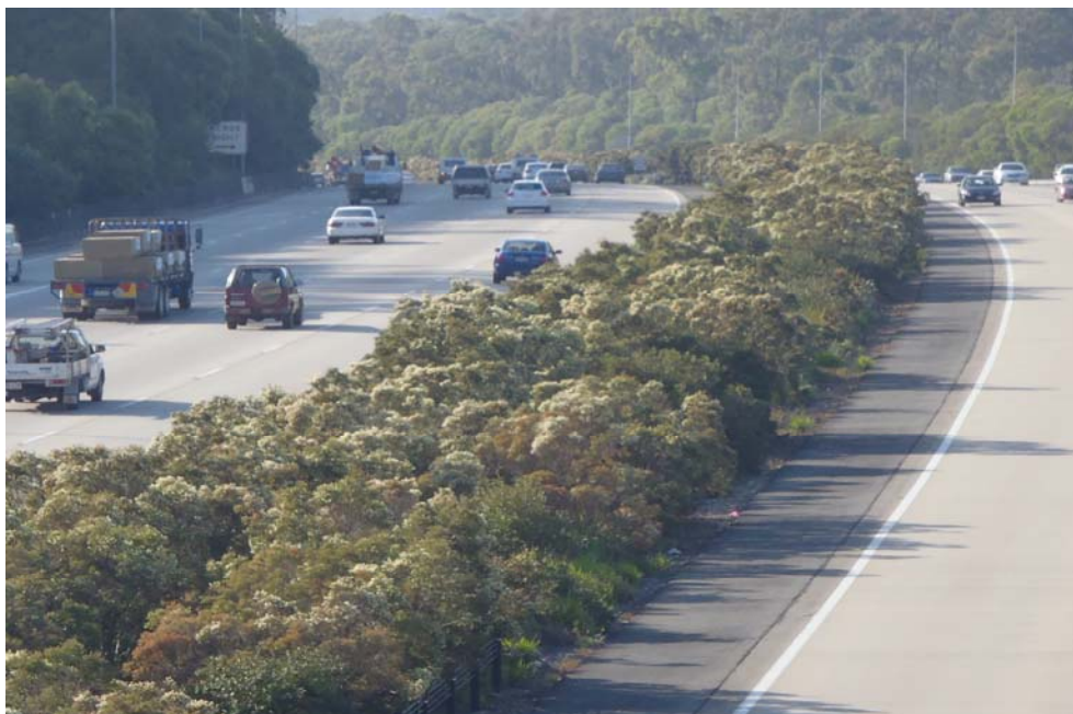
Figure A3-15: The maintenance interventions of planted median will progressively reduce to one intervention per annum
