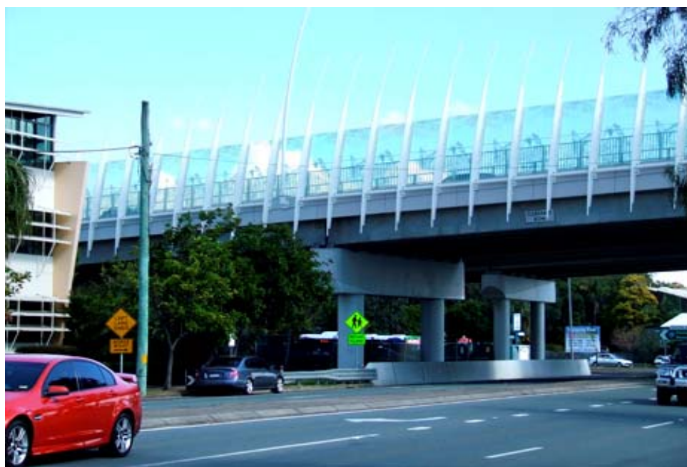
Figure C5-5: Improved surveillance through transparent panels enabling multiple cross views to and from bridge
