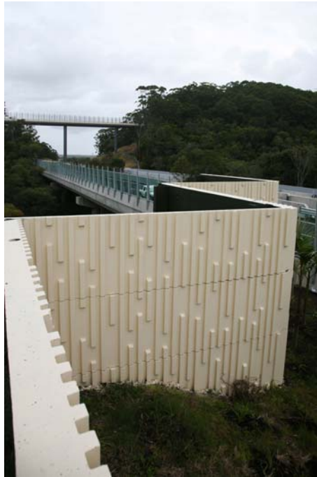
Figure APX2-8: Transparent panels on the bridge are used to retain views where high visual sensitivity was an important community issue
