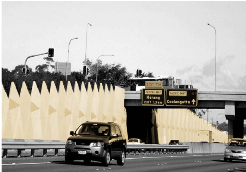
Figure A4-2: Improved legibility through the use of directional patterning in walls and clear signage
