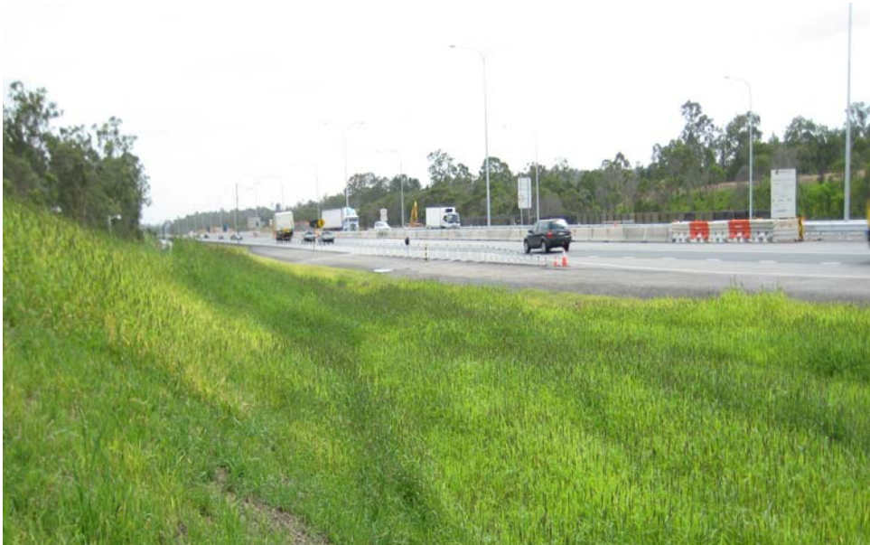
Figure C6-8: Grass seeding used as a temporary erosion and sedimentation control measure during construction
