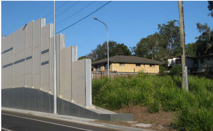
Figure B1-4 Consultation ensures community facilities are designed and implemented to meet council and community requirements
