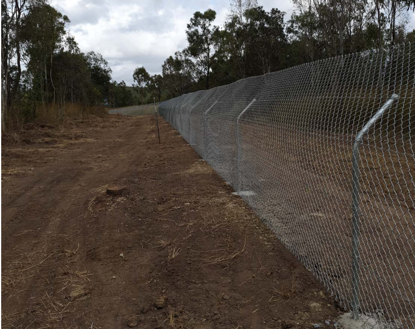
Plate 7: Completed fauna exclusion fencing at Stockyard Creek
