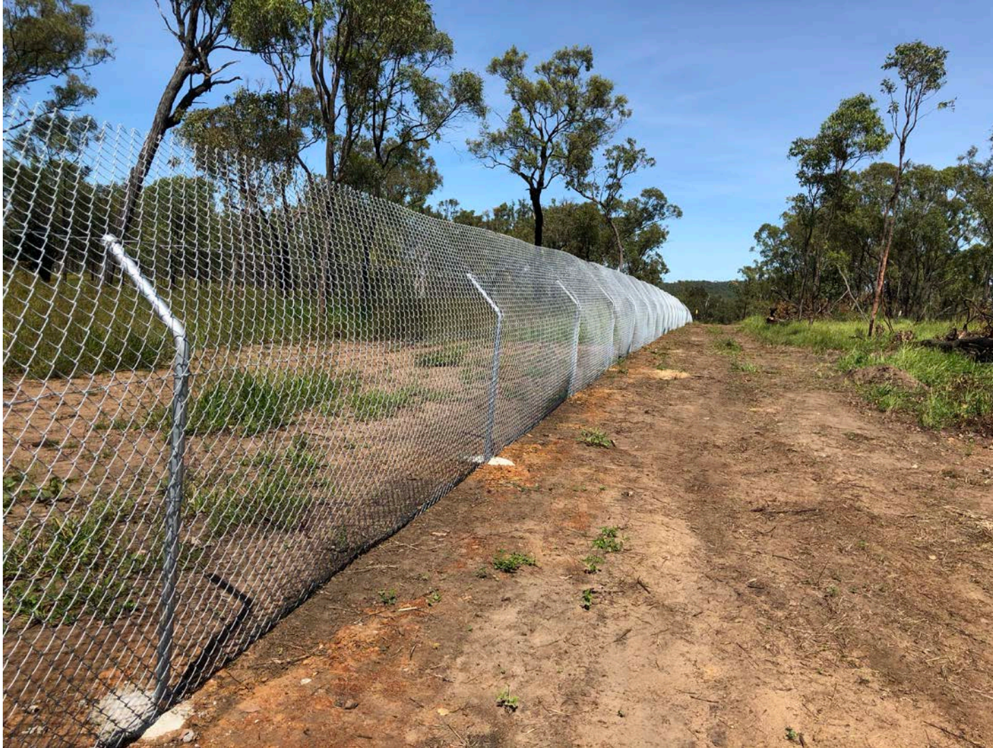
Plate 3: Floppy top fauna fencing design and grubbed fenceline
