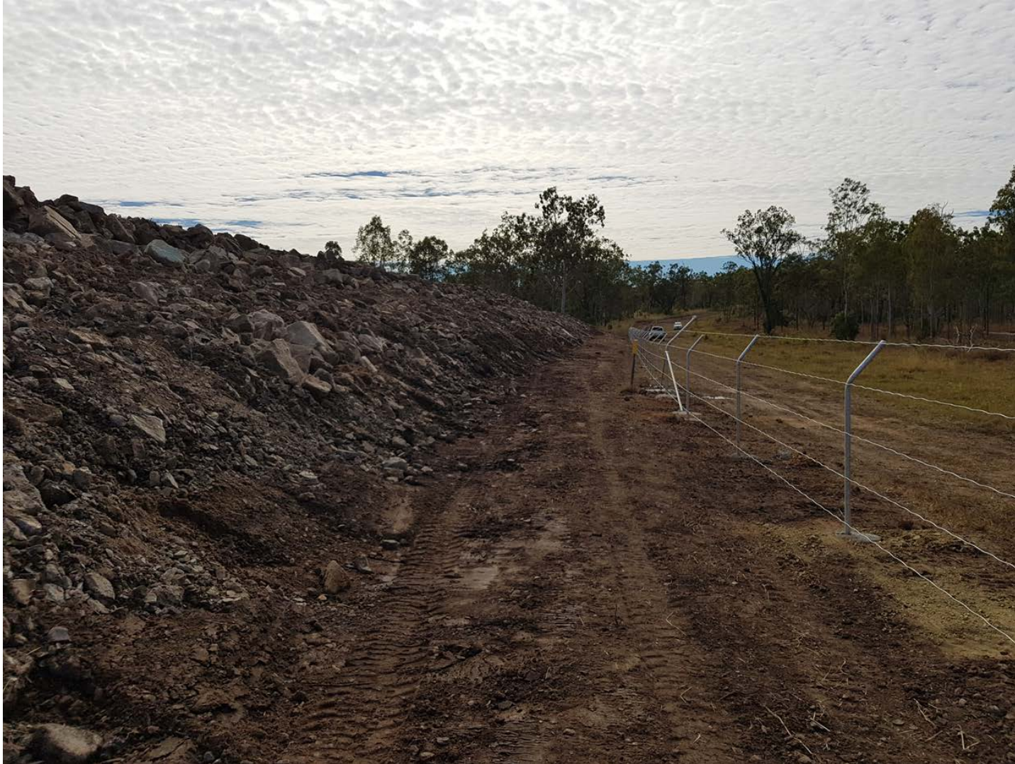
Plate 5: Stockyard Creek fence construction, facing east along the Peak Downs Highway.
