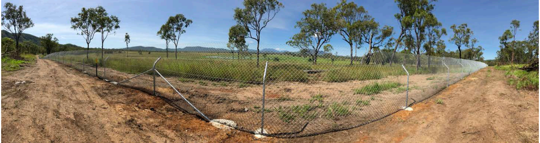
Plate 1: Floppy top fauna exclusion fencing erected immediately north of Denison Creek
