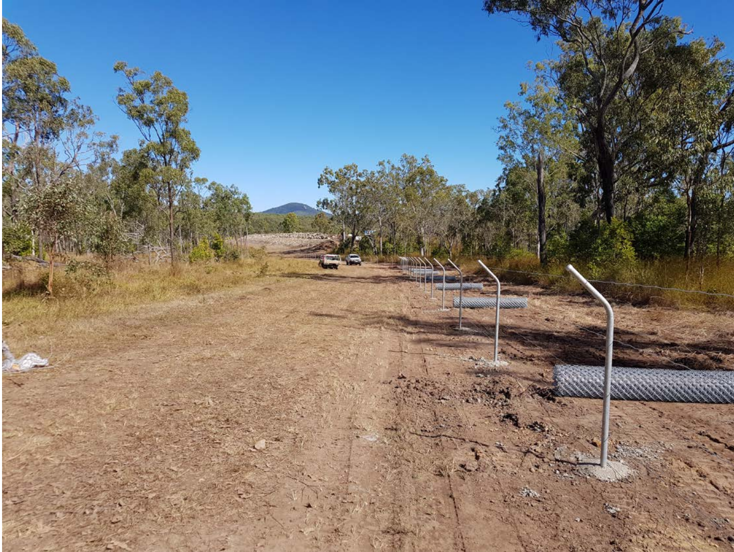
Plate 6: Stockyard Creek fence construction, facing west along the Peak Downs Highway.
