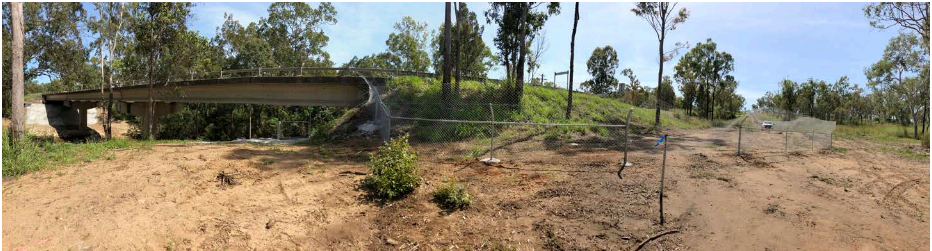
Plate 2: Fencing tied into Denison Creek bridge abutments to provide safe fauna passage
