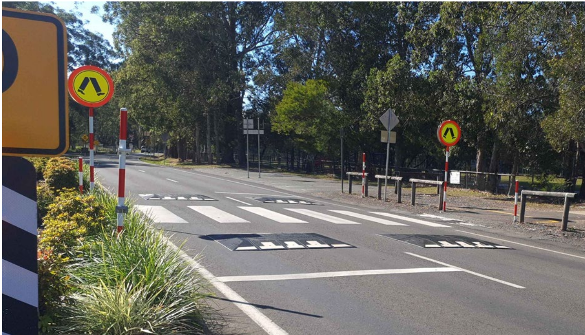
Figure 5.1.2 – Speed cushions reduce vehicle speeds at approaches to zebra crossing
