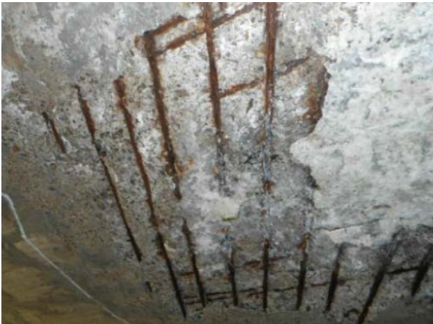
Figure 2.2.4c – Spalling of slab soffit
