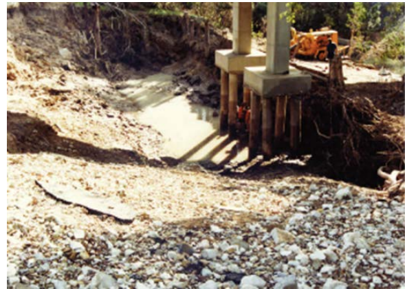
Figure 3.5.7d – Settlement of rigid batter protection
