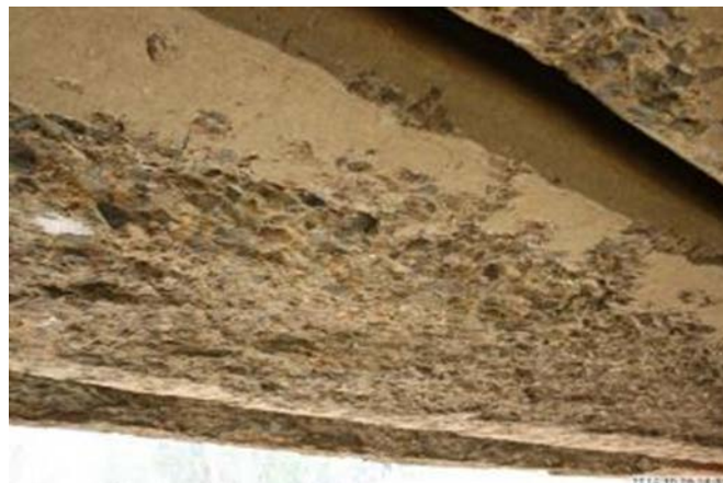
Figure 2.2.7b – Concrete disintegration
