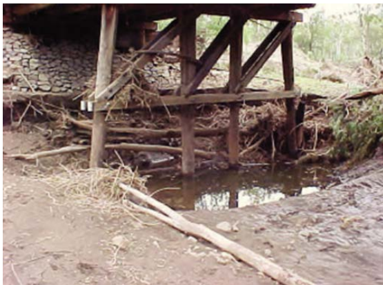
Figure 3.5.7c – Localised scour around pier piles and debris build-up
