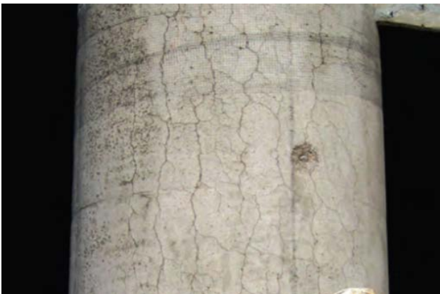
Figure 2.2.2c – Example ASR crack pattern in pier headstock
