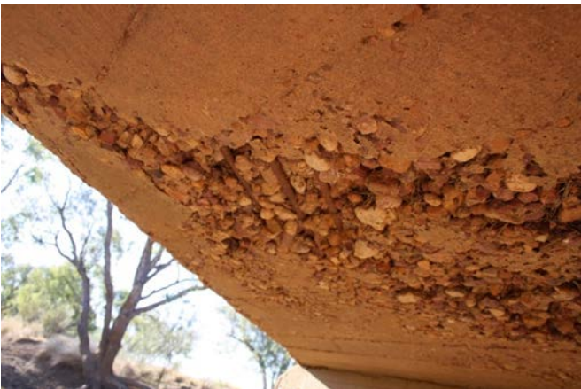
Figure 2.2.6e – Concrete honeycombing
