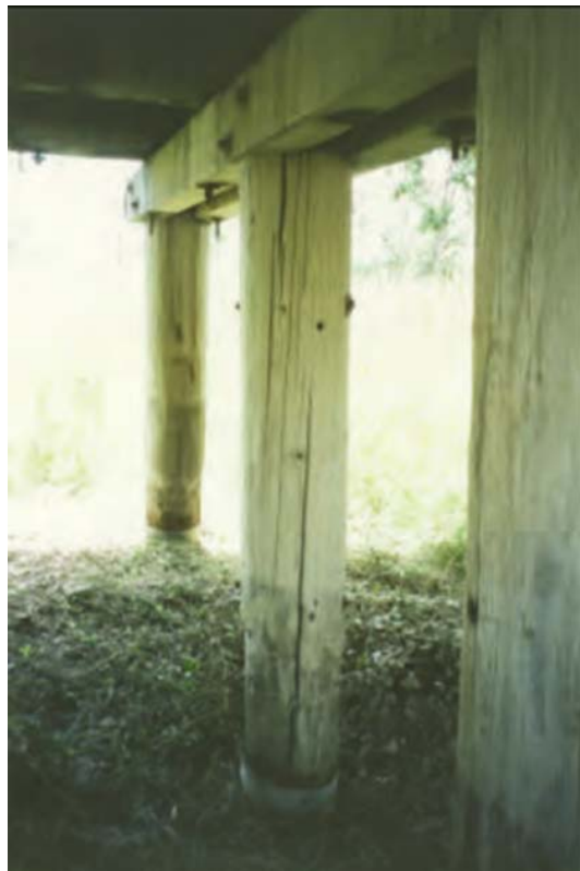
Figure 3.3.5b – Splitting of pile beneath headstock
