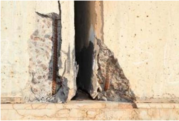
Figure 2.2.4c – Spalling of slab soffit
