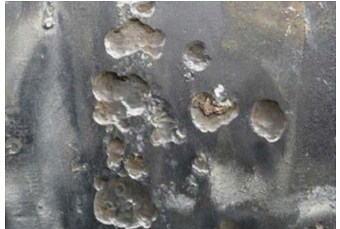
Figure 2.3.1d – Corrosion of steel by SRB
