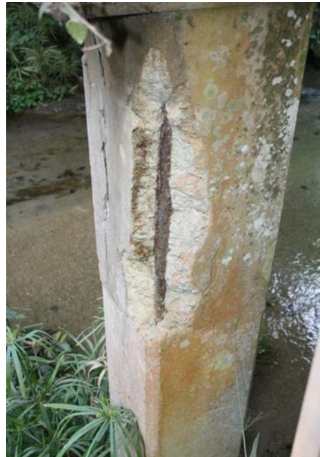
Figure 2.2.4d – Corner spalling of square pile
