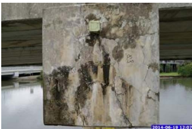
Figure 2.2.2c – Example ASR crack pattern in pier headstock
