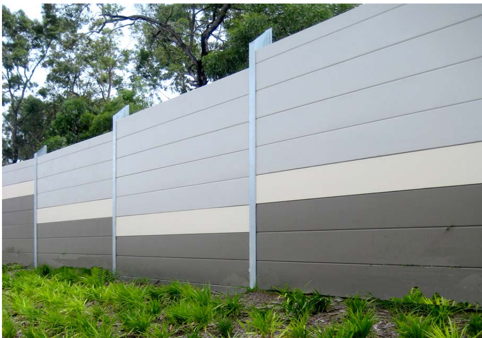
Figure C3-7: Colour and pattern in conjunction with material selection used in noise barriers design to create visual interest and express corridor themes
