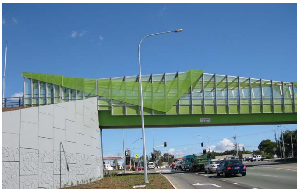
Figure C3-14: Footbridge as a visual feature element within the road landscape with detailed attention to throw screen design
