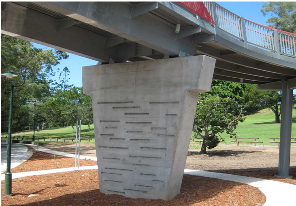
Figure C3-2: Tapered and textured piers create a visually recessive structure within the road landscape
