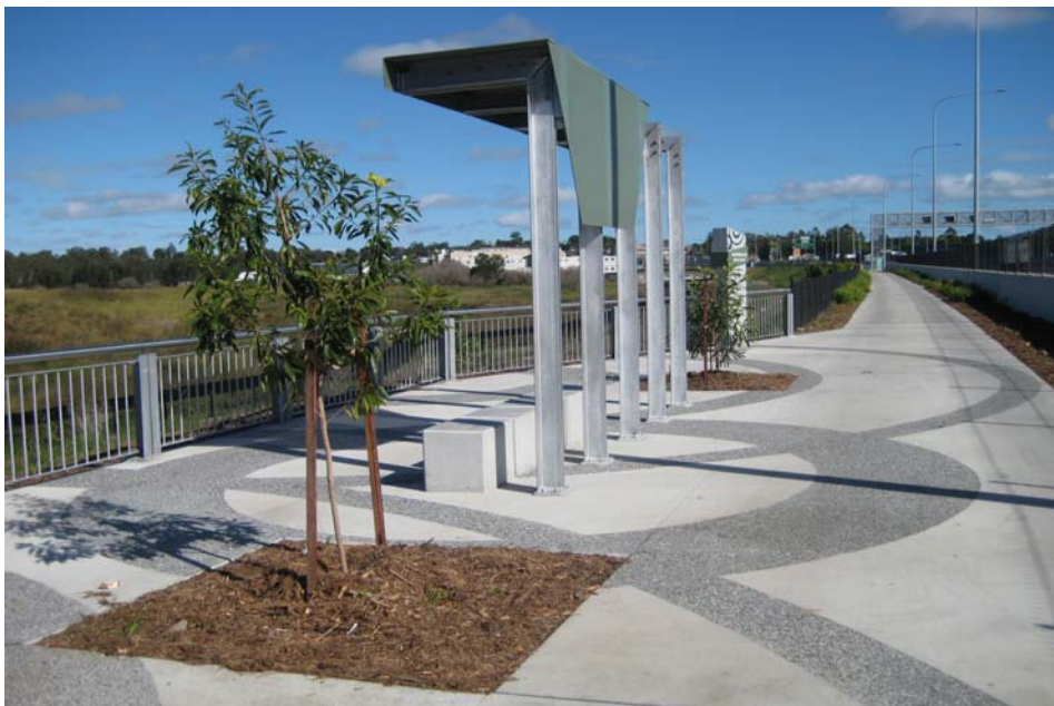
Figure C3-12: Integration of pavement treatments to cycleway facilities
