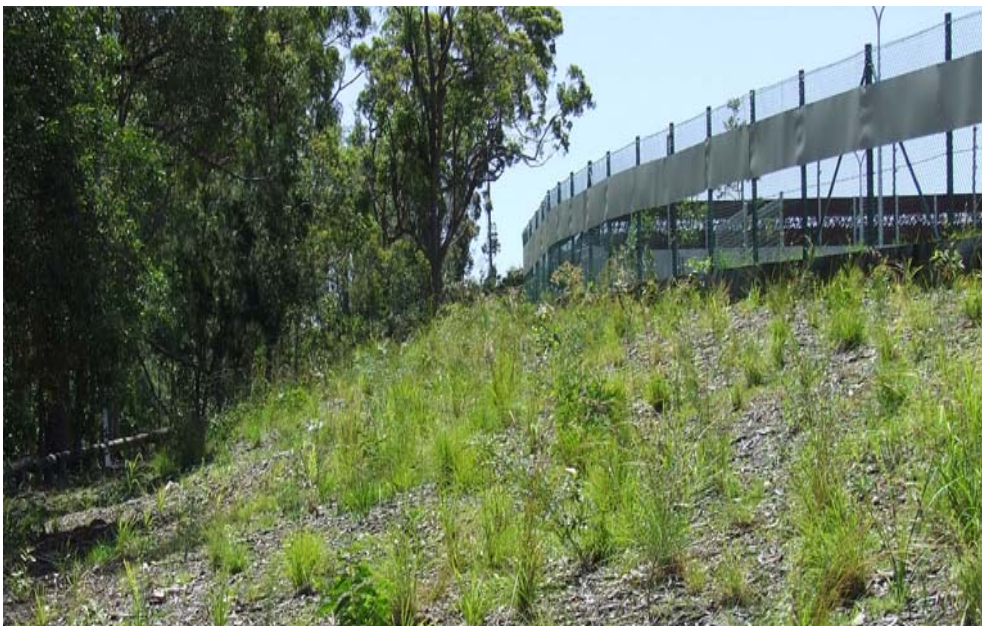
Figure C6-11: Fauna fencing and adjoining landscape treatment limit fauna from accessing roadways
