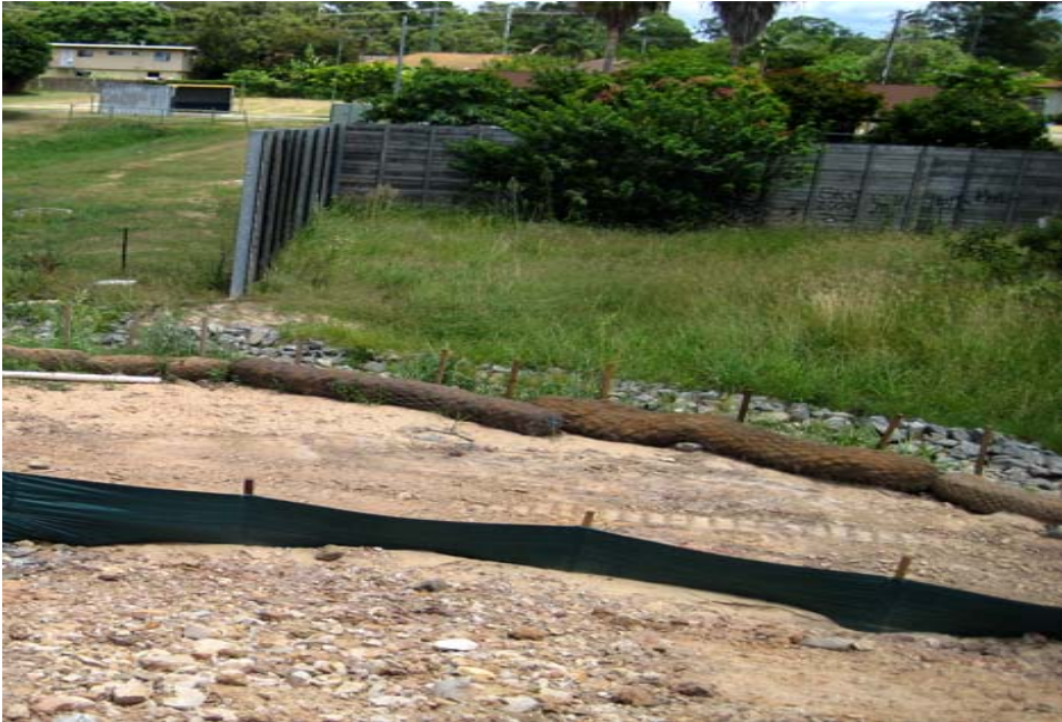
Figure C6-6: Erosion and sediment control measures minimizing construction impacts on adjoining residences
