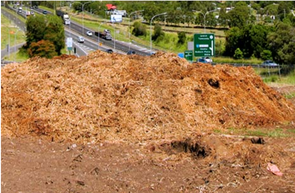
Figure C6-7: Removed local vegetation chipped for use as site mulch
