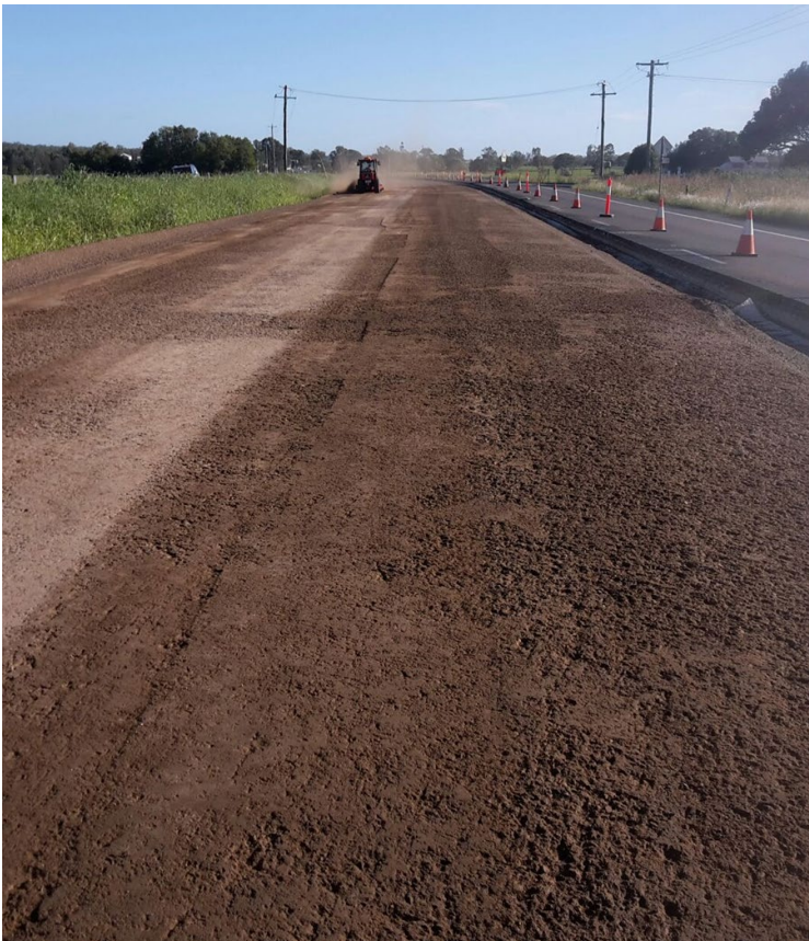
Figure 8.8.9.4.2(b) – Rotary broom removing loose material from a hard-cut surface
