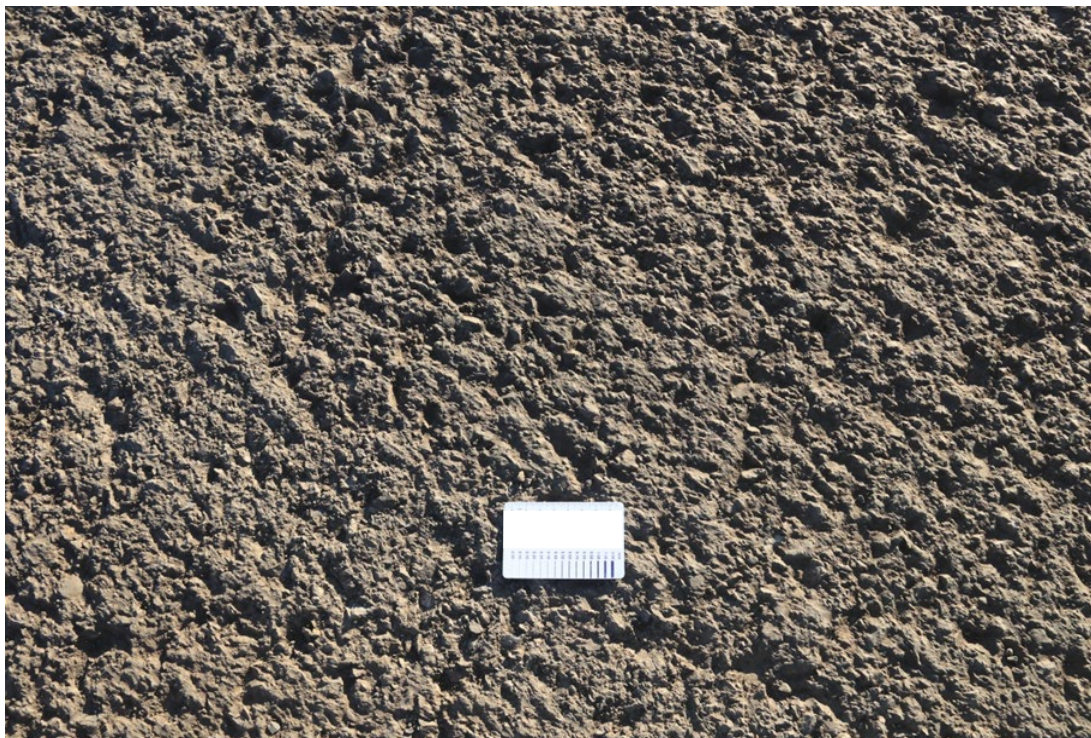
Figure 8.8.9.4.2(c) – Example of an acceptable hard-cut surface
