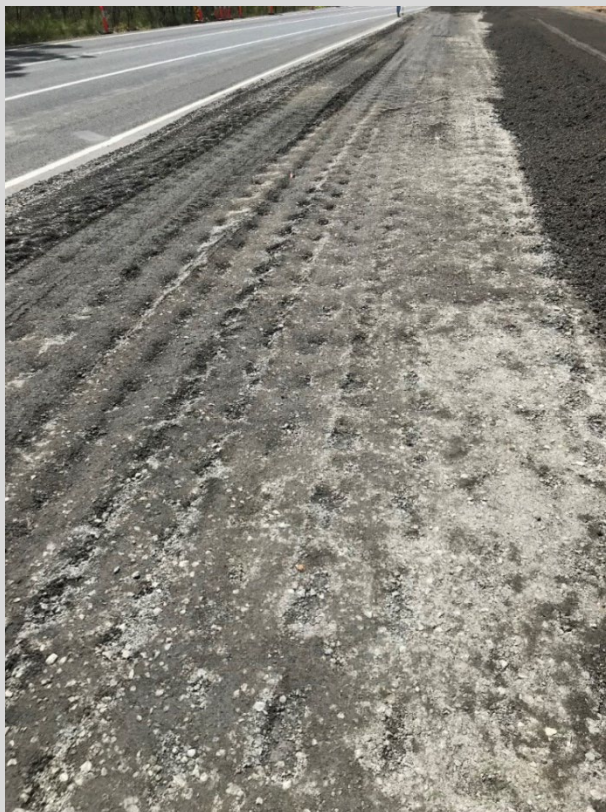
Figure 8.8.9.4.4(b) – Example of an unacceptable padfoot surface that has been “smoothed out” by construction activities
