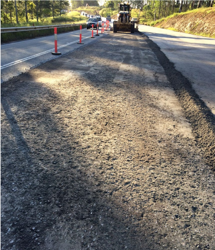
Figure 8.8.9.4.2(a) – Hard-cut of surface with a grader
