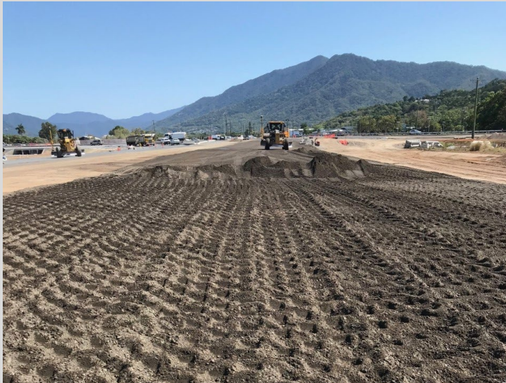
Figure 8.8.9.4.4(b) – Example of an unacceptable padfoot surface that has been “smoothed out” by construction activities
