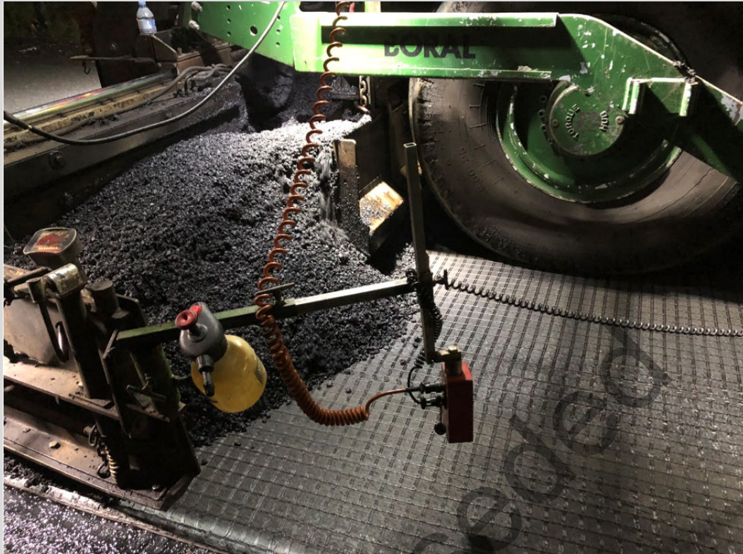
Figure 9.7.1 – Example of asphalt being paved on asphalt geosynthetic with no bow-waves, wrinkles or folds
