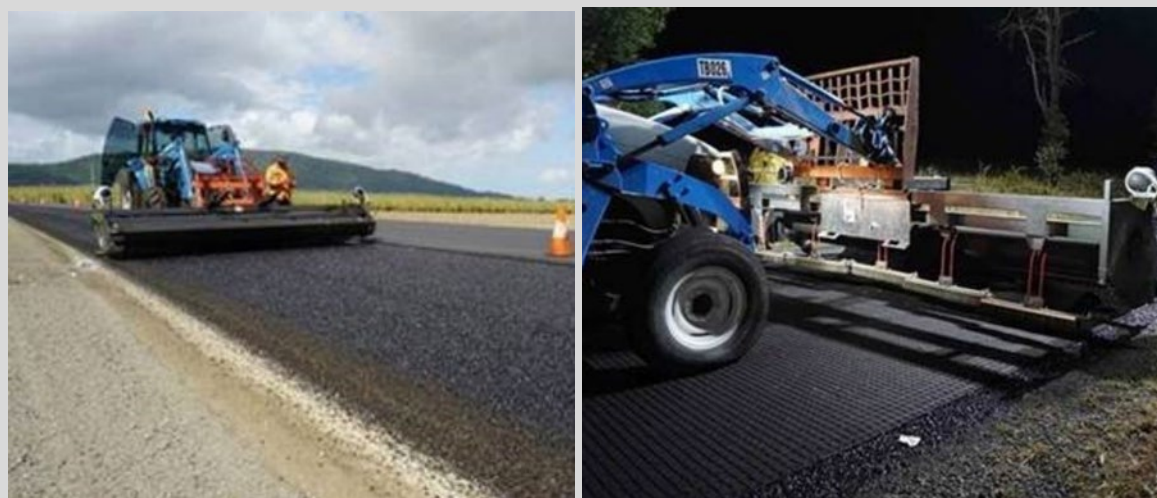
Figure 9.6.2 – Examples of installation of asphalt geosynthetics using application frame
