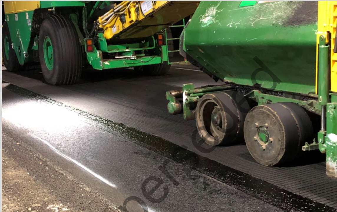
Figure 9.6.3(b) – Example of minimum bitumen pick-up on truck tyres or paving equipment
