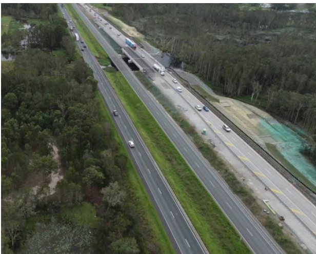
New southbound lanes (far right) between Pumicestone and Caboolture-Bribie Island roads
