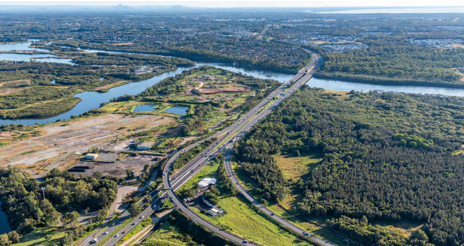
Aerial image of Gateway Motorway and Bruce Highway merge, northbound
