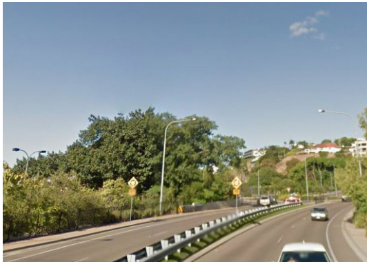
This four lane urban arterial would see TMR responsible for all carriageway from channel to channel.
