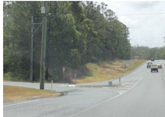
An example of deceleration and acceleration lanes at an intersection. TMR is responsible for the entire carriageway.
