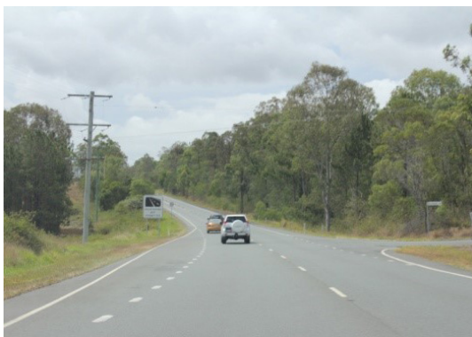
An example of auxiliary lanes at an intersection. TMR is responsible for the entire carriageway.
