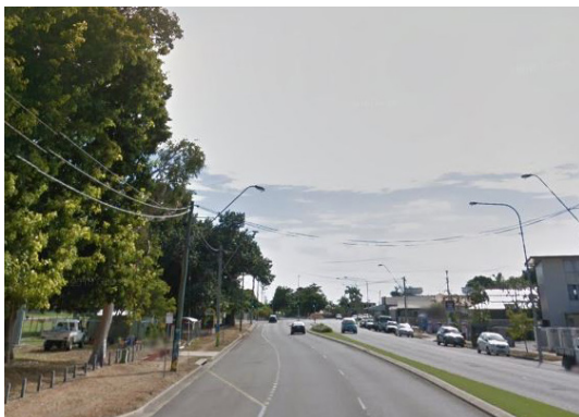
The edge line widening at the bus stop provides demarcation of traffic lanes that are the responsibility of TMR.
