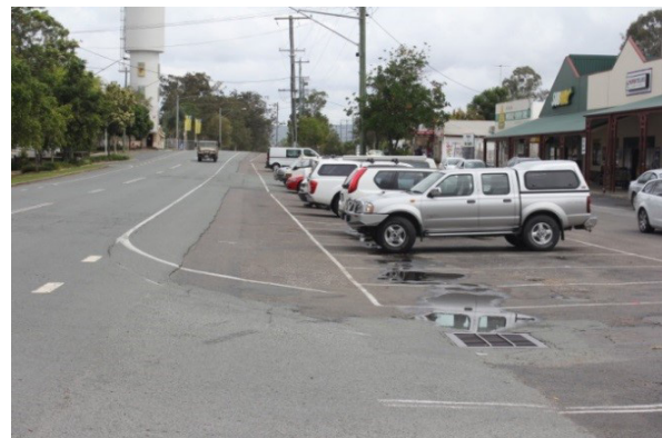
The photo illustrates the limits of asphalt overlay for the shoulder/cycle lane and the demarcation of TMR and Local Government responsibilities.
