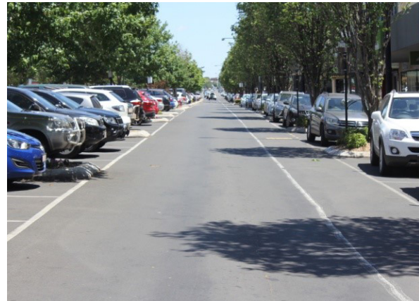
Given this road has a cycle lane and centre parking, TMR is responsible for the traffic lanes and cycle lane with Local Government responsible for that part of the carriageway being used for parallel and centre parking.
