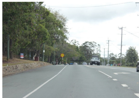
The edge line provides demarcation between the through traffic lane and the parking lane. Responsibilities for parking lanes are discussed in Module 3.
