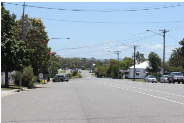
Local Government is responsible for this vast area of carriageway from the outer edge of the cycle lane to the channel.
