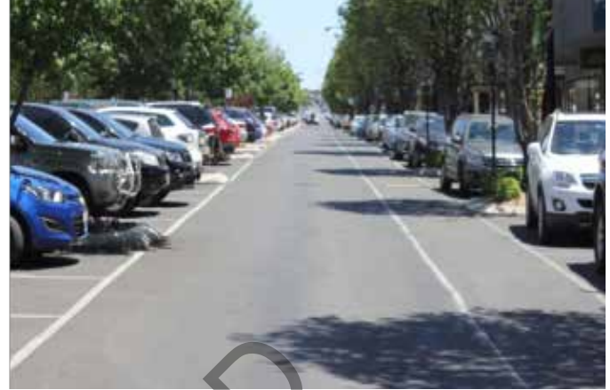
Given this road has a cycle lane and centre parking, TMR is responsible for the traffic lanes and cycle lane with Local Government responsible for that part of the carriageway being used for parallel and centre parking.
