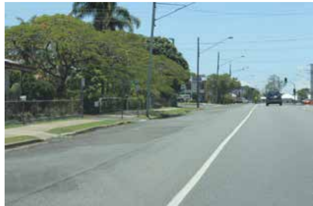
In the case of urban arterials, TMR is to fund the costs of road lighting even though there will be some spillage from road lighting that illuminates the footpath for pedestrians.
