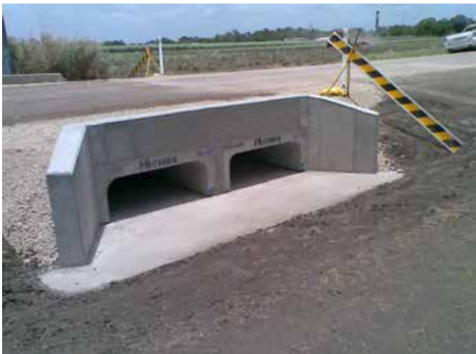
TMR is responsible for road culverts on SCR carriageways.
