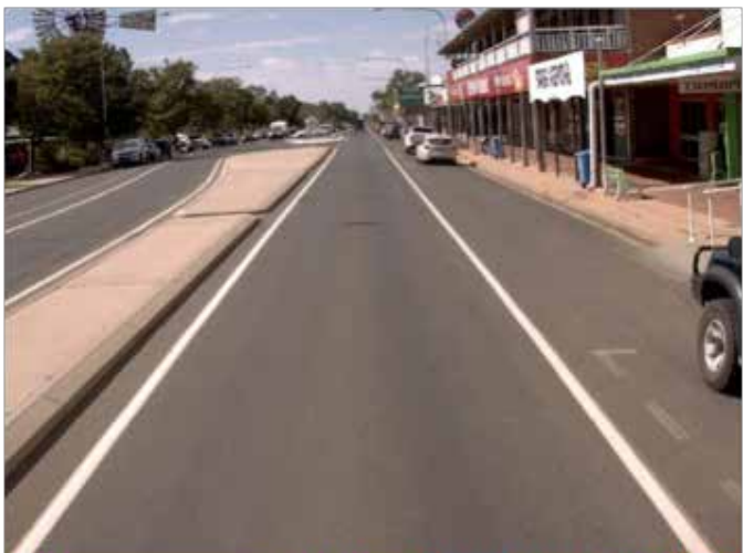
Given the minimum widths of shoulder or cycle lane, Local Government is responsible for a narrow section of parking lane from the outer edge of the shoulder/cycle lane to the channel. To avoid the inefficiencies of both TMR and Local Government undertaking rehabilitation or reseals, a cost sharing agreement should be negotiated so the entire carriageway works can be undertaken at the same time.
