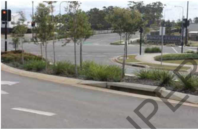
TMR is responsible for the stand-alone sub-surface drainage (gullies, manholes, inlets, outlets) of an intersection on the SCR where the sub-surface stormwater drainage is not connected to Local Government's stormwater drainage network.
