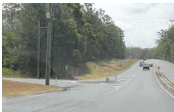
An example of deceleration and acceleration lanes at an intersection. TMR is responsible for the entire carriageway.
