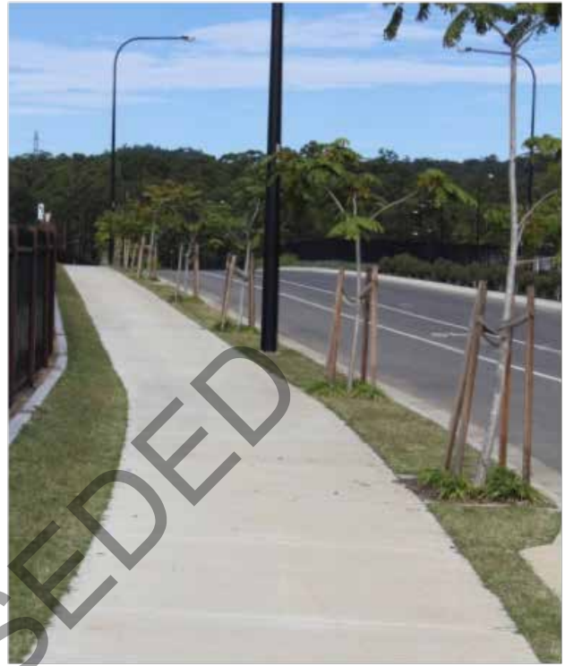
Local Government is responsible for the area (including footpath) from the back of kerb to the property alignment.
