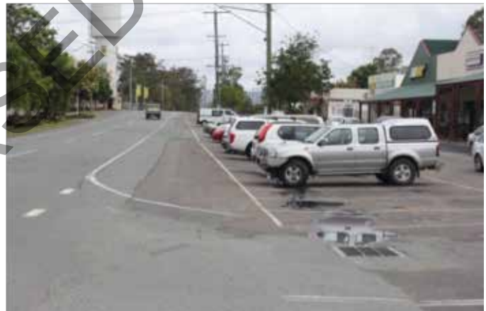
The photo illustrates the limits of asphalt overlay for the shoulder/cycle lane and the demarcation of TMR and Local Government responsibilities.
