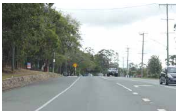
The edge line provides demarcation between the through traffic lane and the parking lane. Responsibilities for parking lanes are discussed in Module 3.
