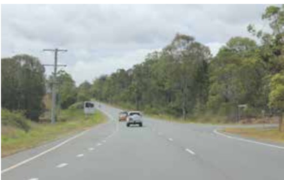
An example of auxiliary lanes at an intersection. TMR is responsible for the entire carriageway.
