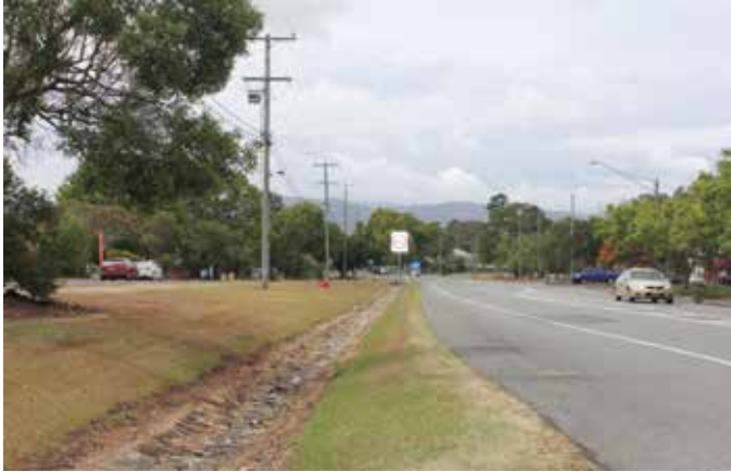
TMR is responsible for maintenance of the rock lined/concrete lined table drain.
