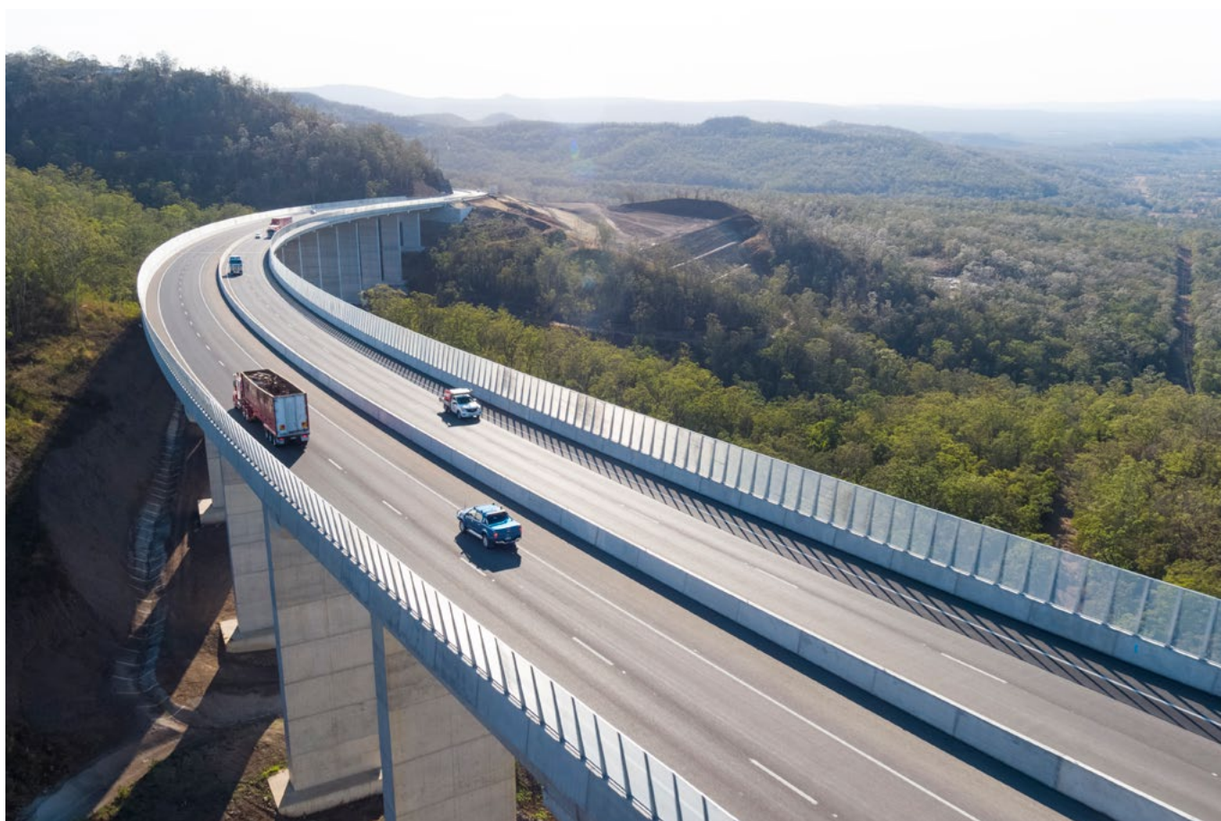
Toowoomba Bypass viaduct
