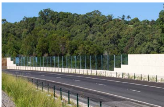
Figure 7.5.4 - Retaining view of high scenic value using transparent barriers
