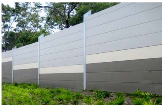
Figure 7.7 (c) - Preserving horizontal lines on uneven ground
