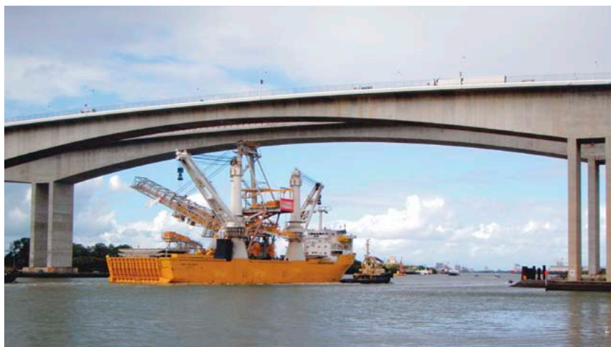
Cargo ship travelling beneath the Gateway Bridge
