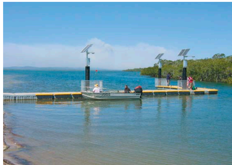
Maaroom pontoon facility
