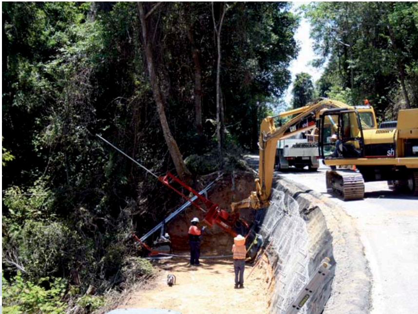
Soil nailing gun being prepped for use on the Kuranda Range
