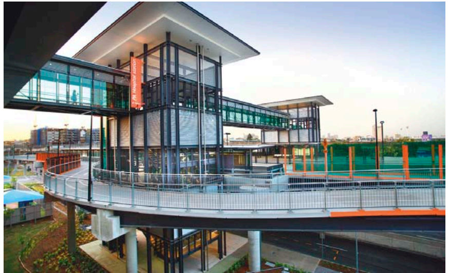
Boggo Road Busway station
