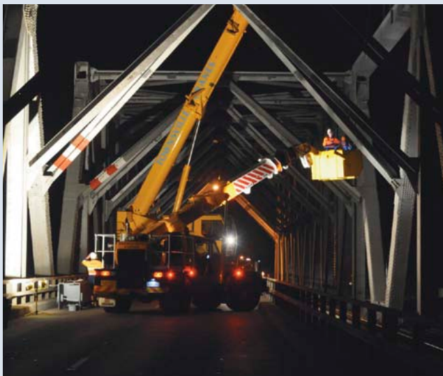
Night work on the Burdekin Bridge
