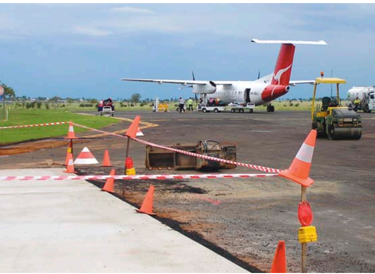
Roma – work in progress on the Apron upgrade
