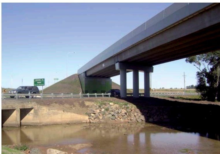
Bundaberg Ring Road
