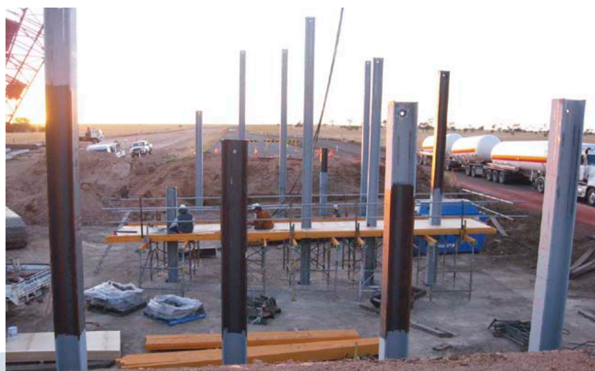
Construction on the Kynuna Bridge
