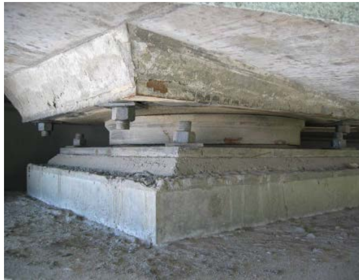
Figure 2 – Sliding pot bearing
