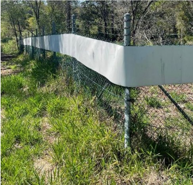
Figure 3.4(a) – Combined security and koala-exclusion fencing with barbed wire at Dholes Rocks Road in Brisbane is a risk to flying-foxes, birds and gliders
