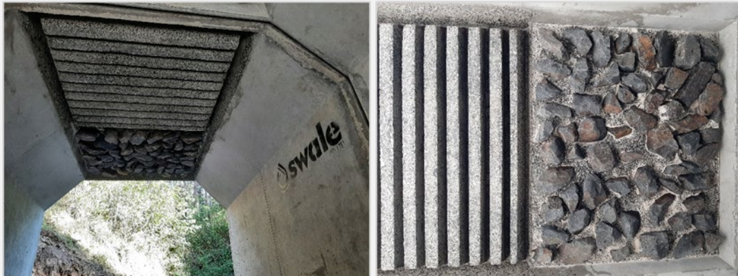
Figure 6.3(c) – The ceiling of a trial culvert with three different types of pre-cast roosting habitat for microbats
