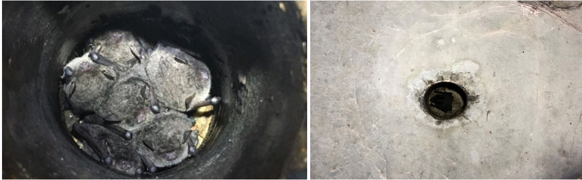
Figure 2.3(a) – Microbat roosts in lift holes
