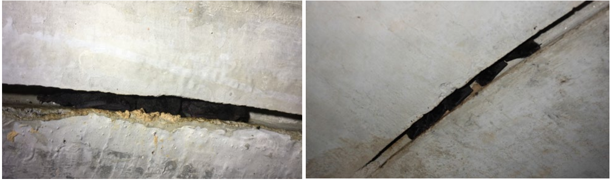
Figure 2.3(c) – Microbat roosts in seals in culverts
