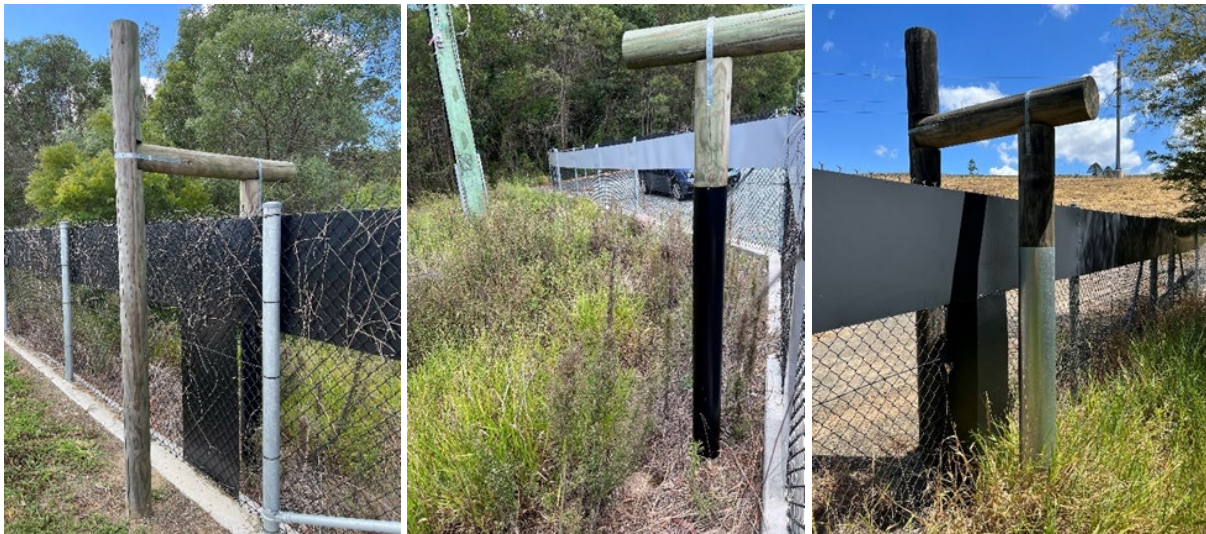
Figure 6.2.2.1 – ‘n-shaped’ koala escape poles
