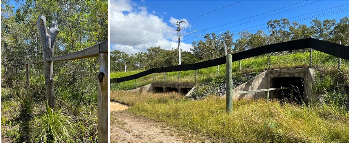
Figure 6.4(a) – Free standing log rails leading to an underpass (left) and through a culvert (right)
