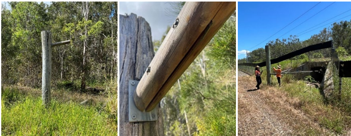
Figure 6.3 – Koala refuge poles made from salvaged tree trunks (left), recycled telephone pole (middle), and treated pine post at end of a horizontal rail (right)
