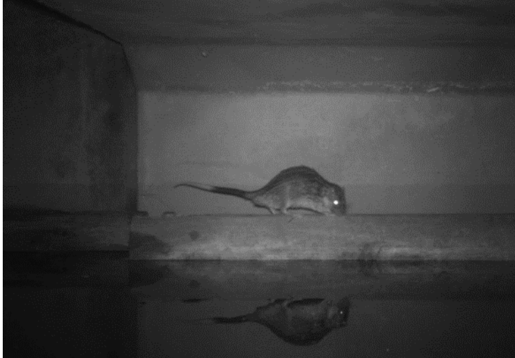
Figure 6.1 – Rakali using the log ledge in an inundated box culvert
