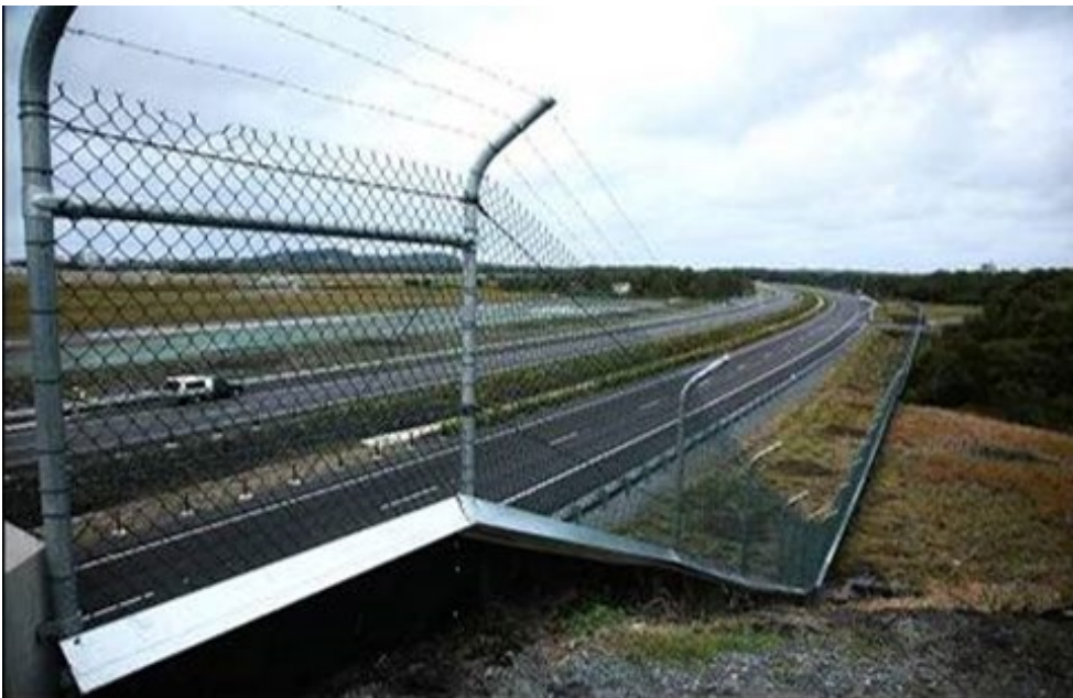
Figure 6.2(b) – Frog fencing attached to security fence
