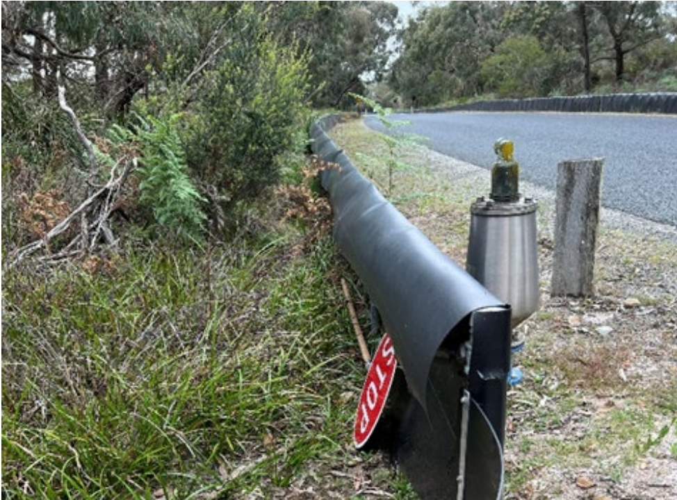
Figure 6.2(a) – Permanent fencing for amphibians showing the overhanging lip that prevents them from climbing over
