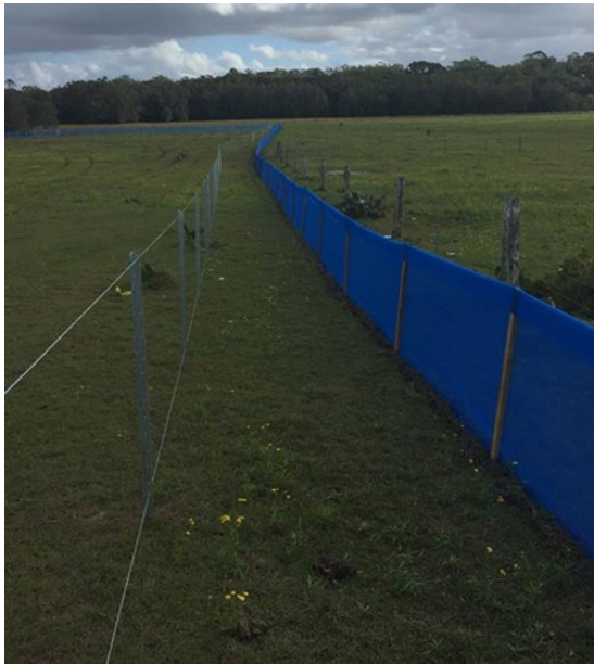
Figure 7.1 – Temporary frog fencing used during construction projects
