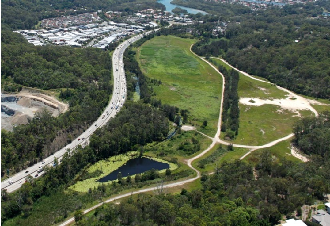
Figure 7(h) – Oyster Creek in 2017 prior to construction commencing
