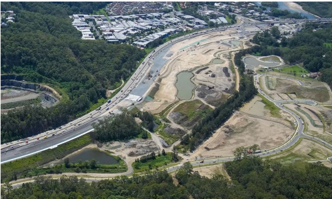
Figure 7(i) – Oyster Creek during construction (March 2023)
