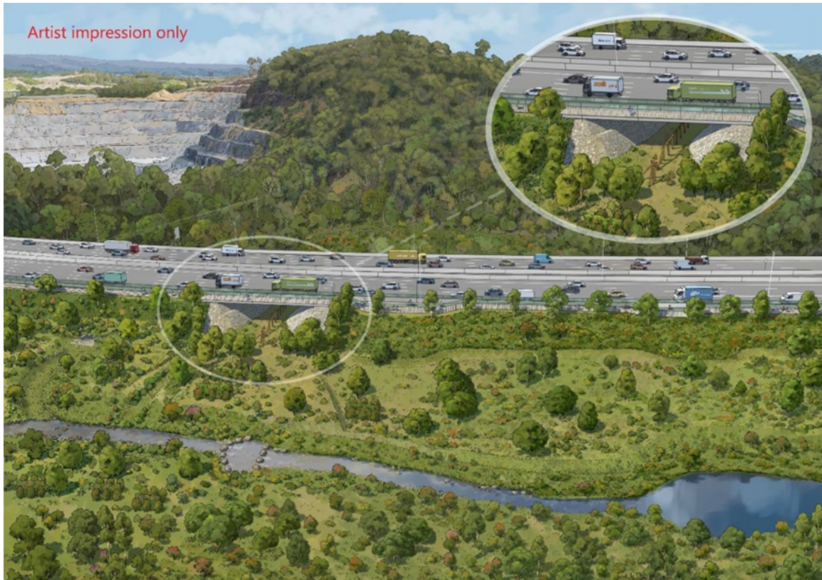
Figure 7(a) – Artist impression of fauna underpass on Burleigh to Palm Beach upgrade of the Pacific Motorway
