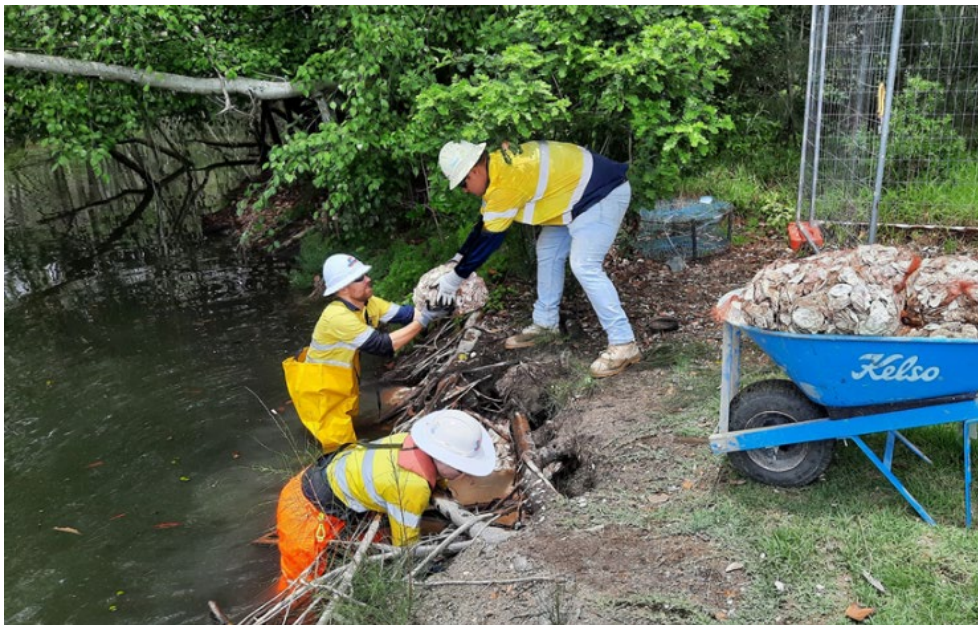
Figure 6.11(a) – Installing biodegradable mesh bags for streambank erosion protection
