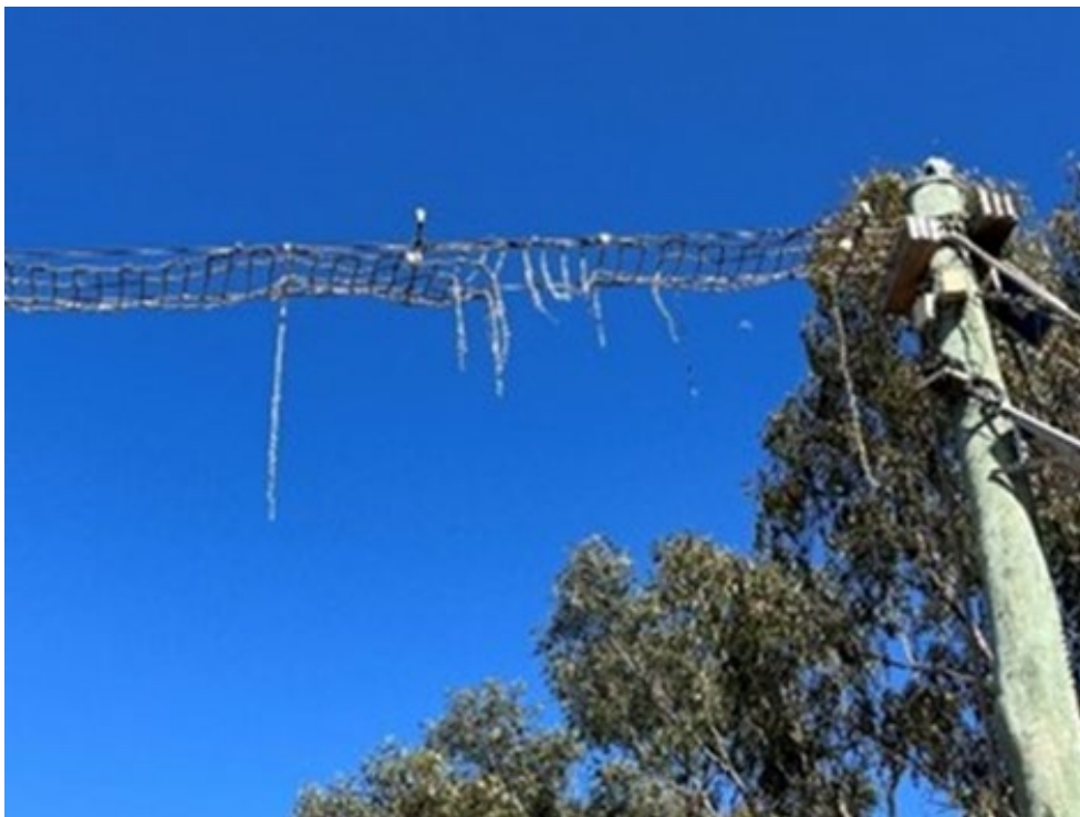
Figure 7(e) – Degradation of rope ladder canopy bridge due to exposure to UV light
