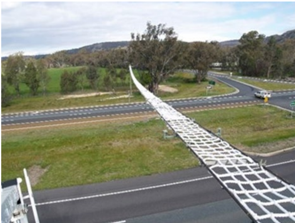
Figure 7(a) – Rope ladder canopy bridge with a 70 metre span across the Hume Freeway, Victoria
