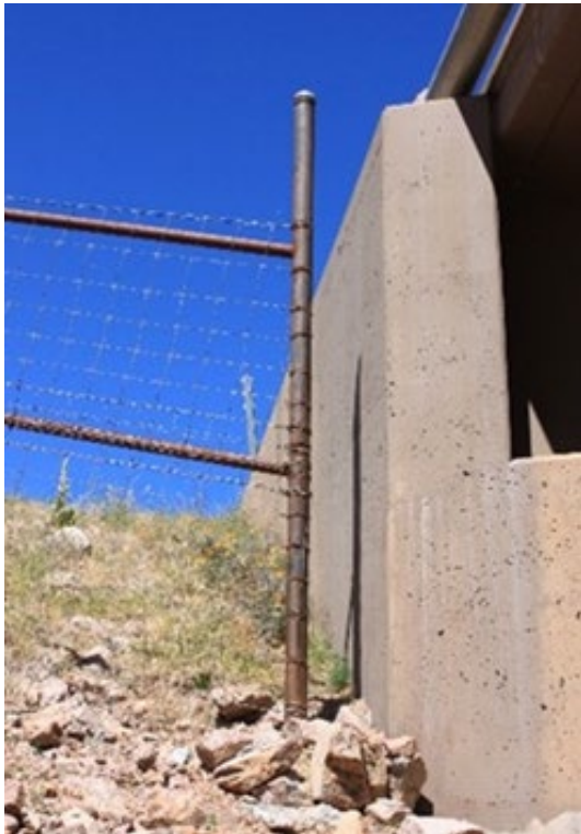
Figure 3(a) – Fencing should be attached closely to crossing structures and other permanent structures to prevent animals squeezing past
