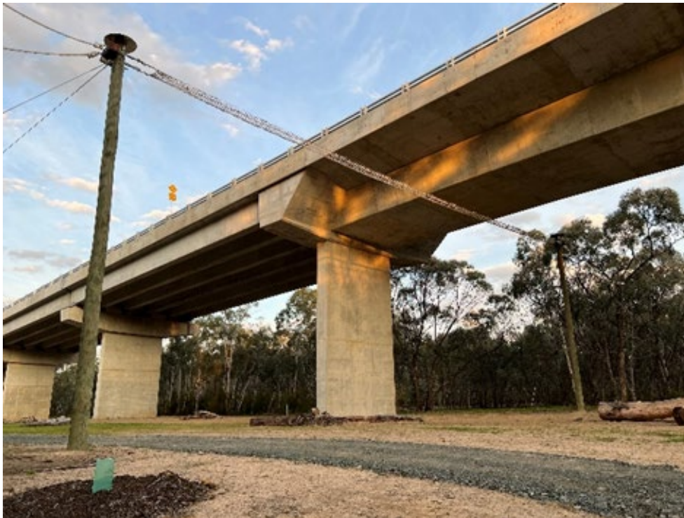
Figure 8(b) – Under-road canopy bridge under the Echuca-Moama bridge in NSW
