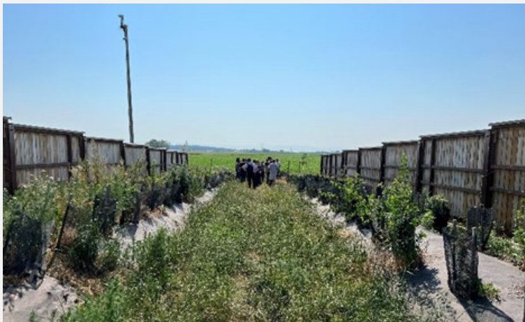
Figure 6(b) – Recently constructed vegetated land bridge in France, with zones and plantings for different species of fauna
