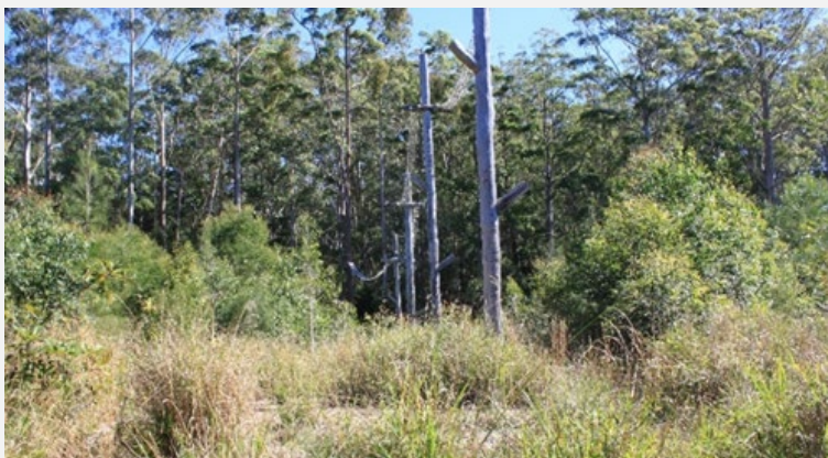
Figure 6(c) – Land bridge over Hamilton Road, Brisbane, showing zones with tall trees and central zone with shorter grasses for different species of fauna
