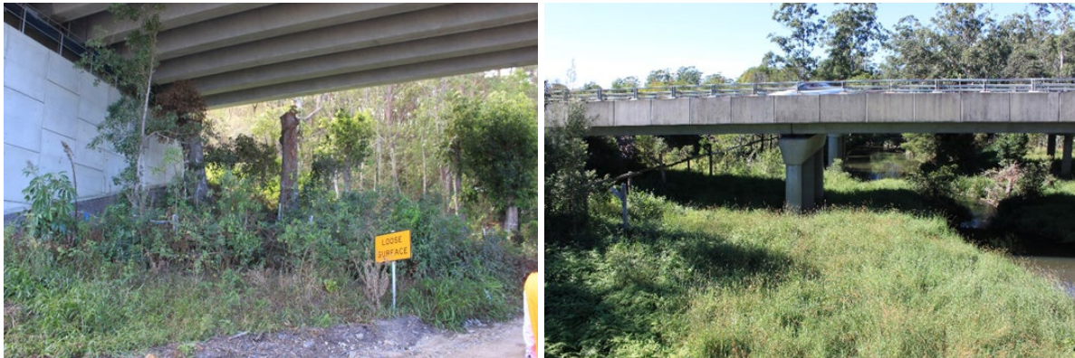
Figure 3(b) – Bridge underpass at the Richmond River on the Pacific Highway, northern New South Wales (left), and Bridge underpass with wide terrestrial fauna zone and koala log rail (right).
