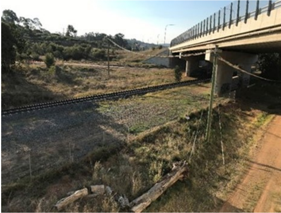
Figure 7(d) – Rope ladder canopy bridge across railway at Kapooka near Wagga Wagga, NSW
