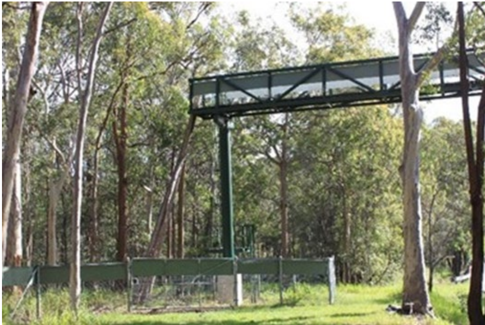
Figure 7(c) – Steel gantry for koalas across Burbank Rd at Mount Cotton, Brisbane
