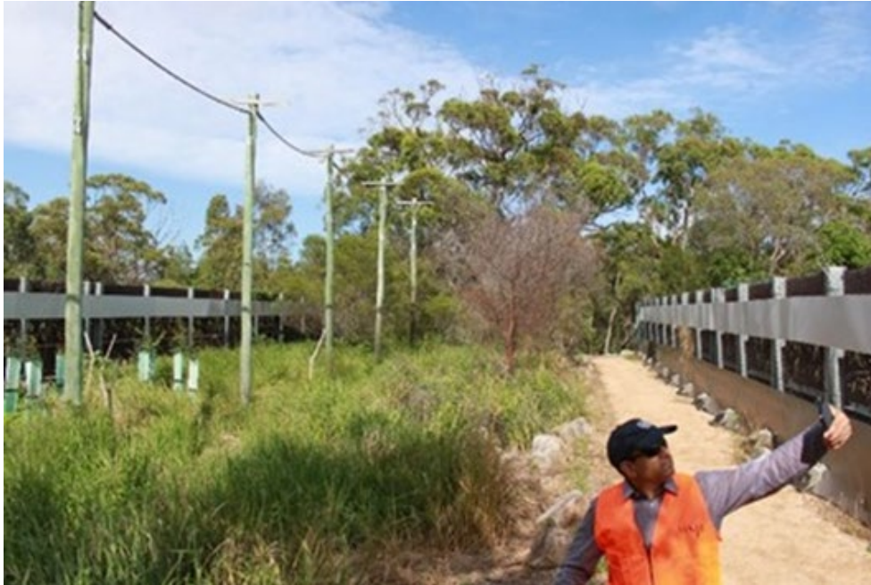
Figure 7(b) – Single-rope canopy bridge on the shared-use land bridge over Hamilton Rd, Brisbane
