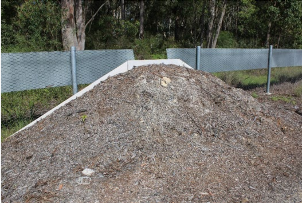
Figure 15.2(a) – Escape ramp on the Woolgoolga to Ballina section of the Pacific Highway
