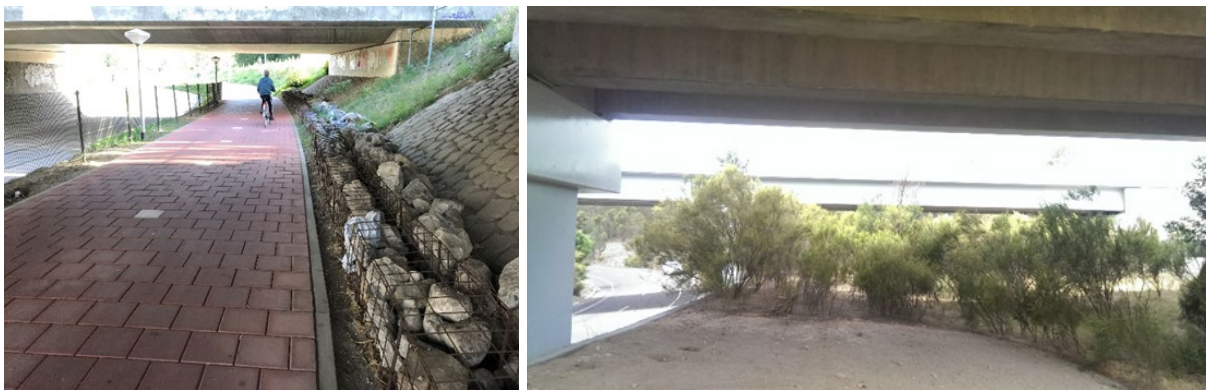
Figure 3(c) – Bridge underpass in The Netherlands, with rock gabion wall for reptile movement (left), and Bridge underpass on the Calder Freeway, Victoria, showing terrestrial fauna zone adjacent to a secondary road (right).
