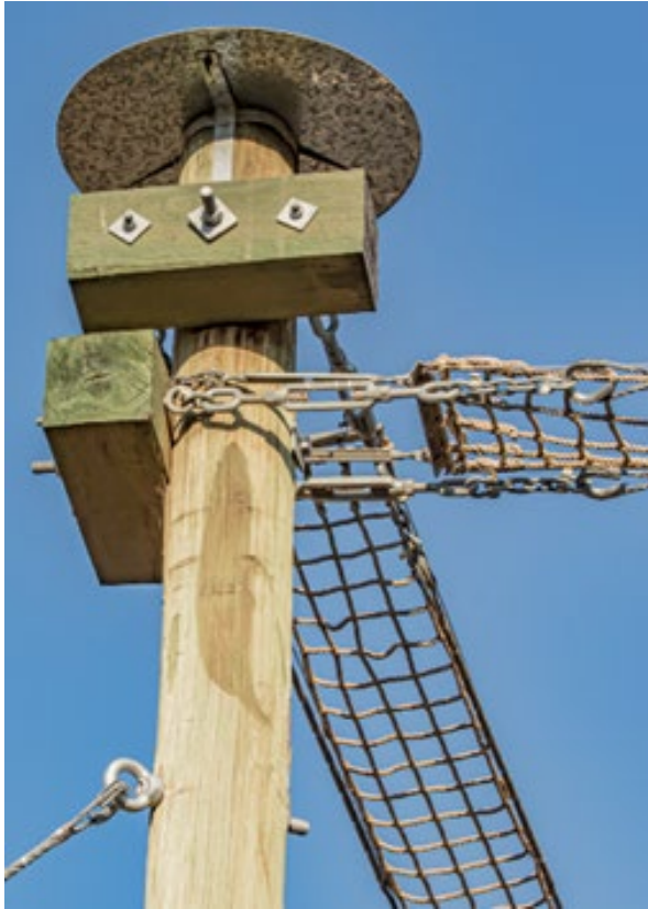
Figure 7(h) – Close-up of timber beams to which the steel cables and rope ladder is attached to
