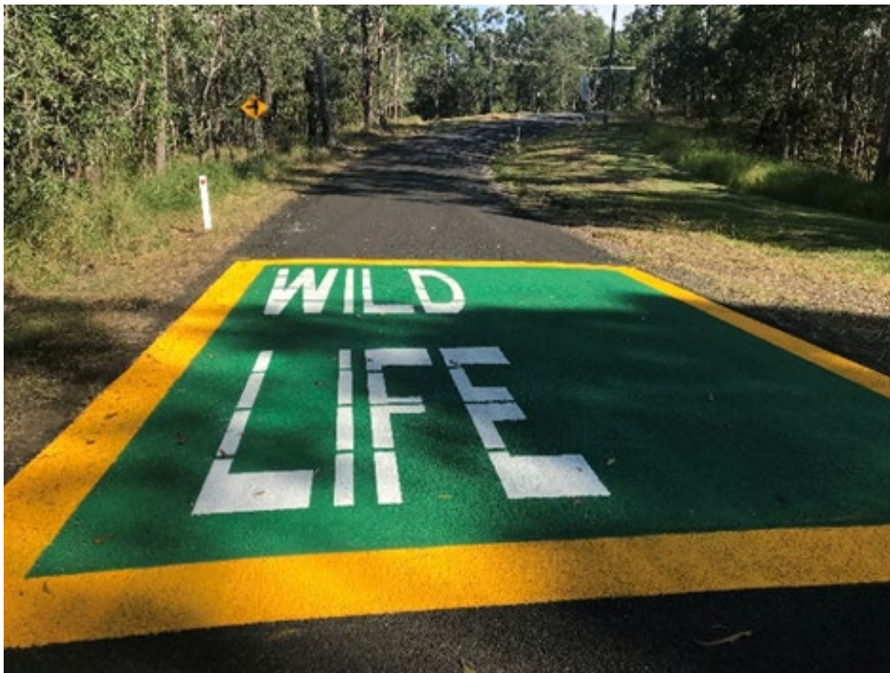
Figure 19.7(c) – Road stencilling in Brisbane warning motorists of the risk of WVC
