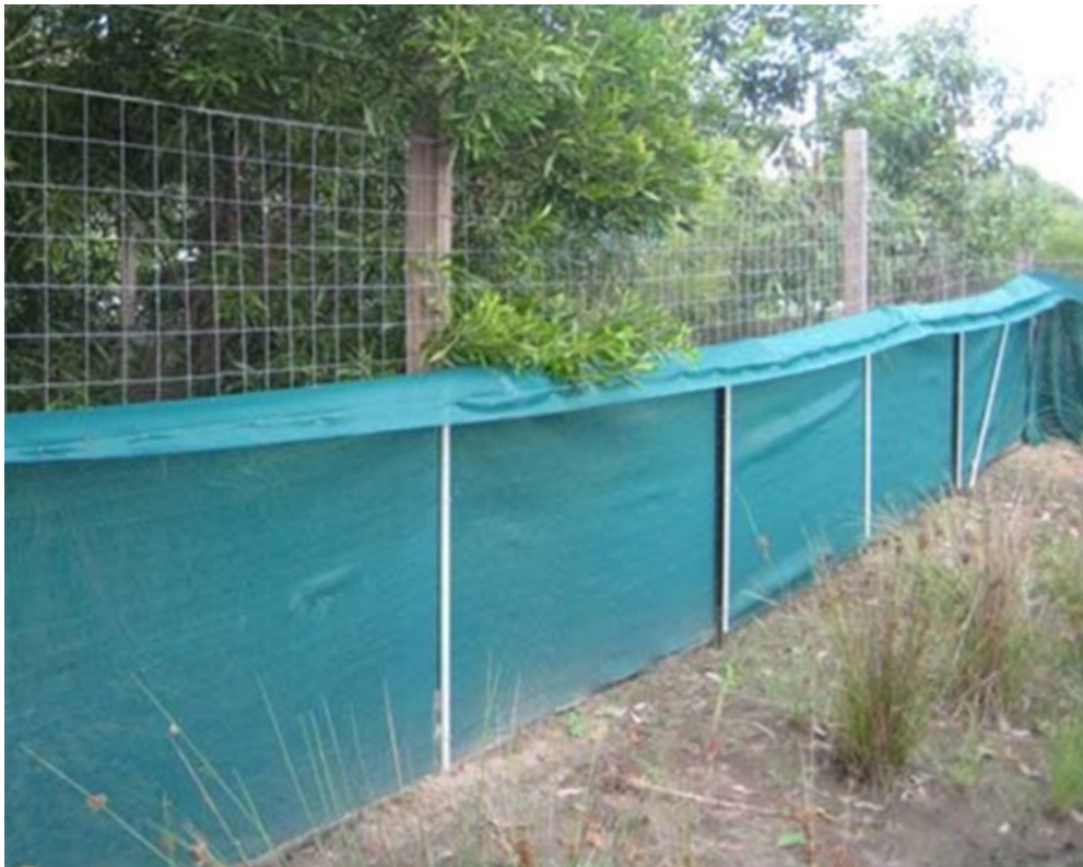
Figure 5.3.3(b) – Temporary fence for amphibians, made of silt fencing
