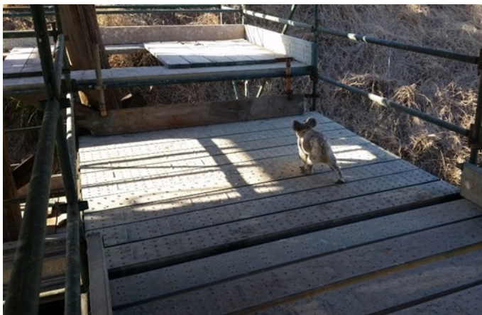
Figure 8.2(b) – Koala and joey leaving site of bridge rehabilitation works.
