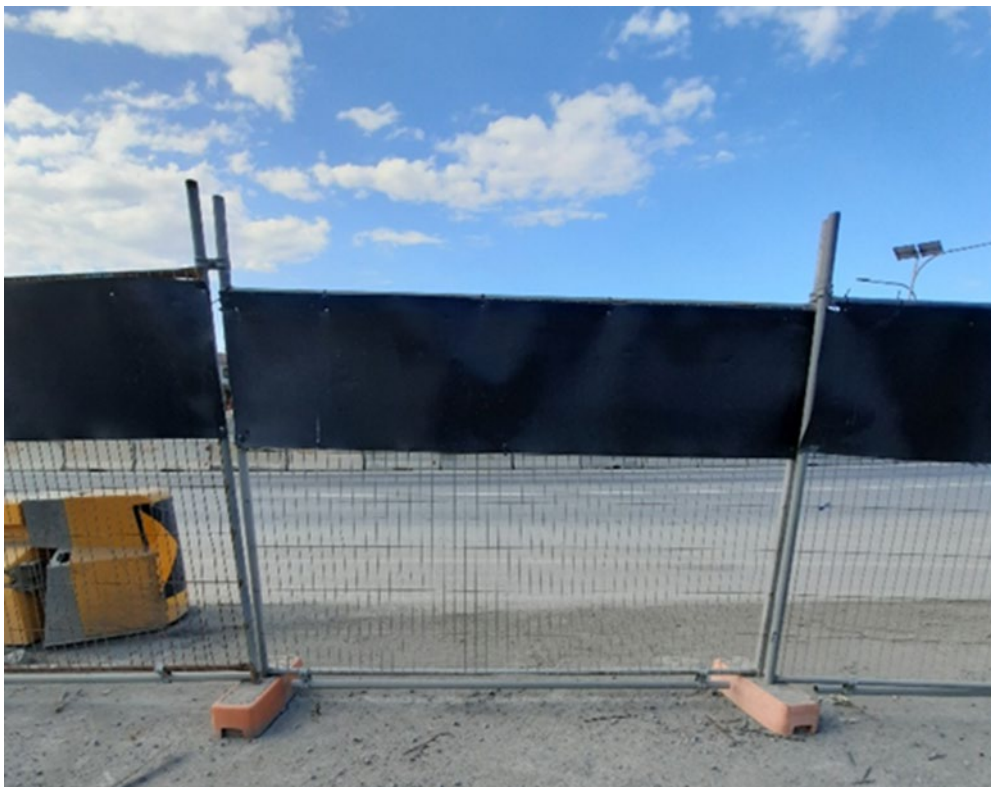
Figure 5.3.3(c) – Plant-hire fencing with panel at top to inhibit climbing by koala
