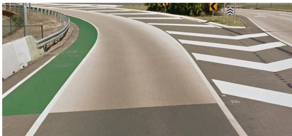
Figure 1 – Typical HFST on a tight curve
